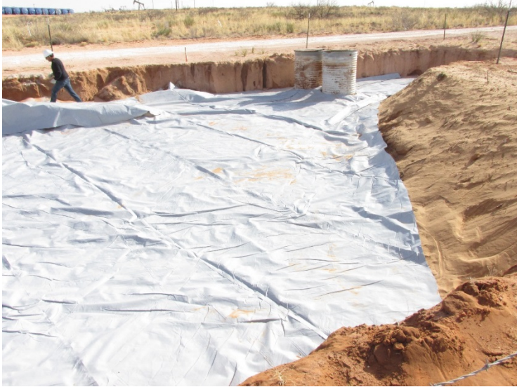
Installation of liner 3/18/14
