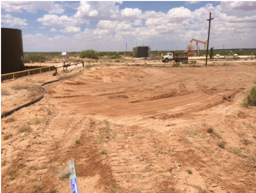
Photograph of backfilling activities at the JRU #124H Tank Battery Release Site.
