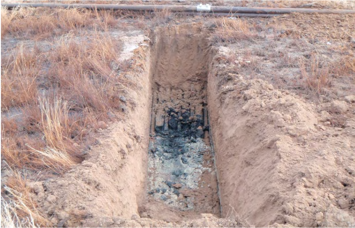
Bass 3 Federal Well #4 Spill Site "B" - Delineation Trench
