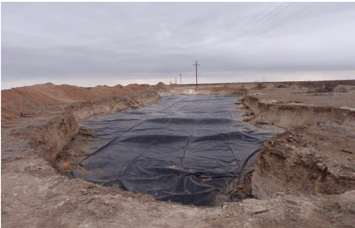
Bass 3 Federal Well #4 Spill Site "B" - Liner Installation
