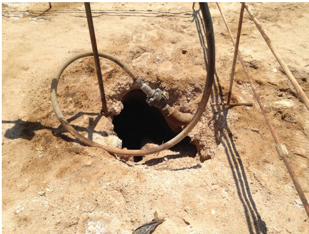
Photo 1. Injection well release point.
