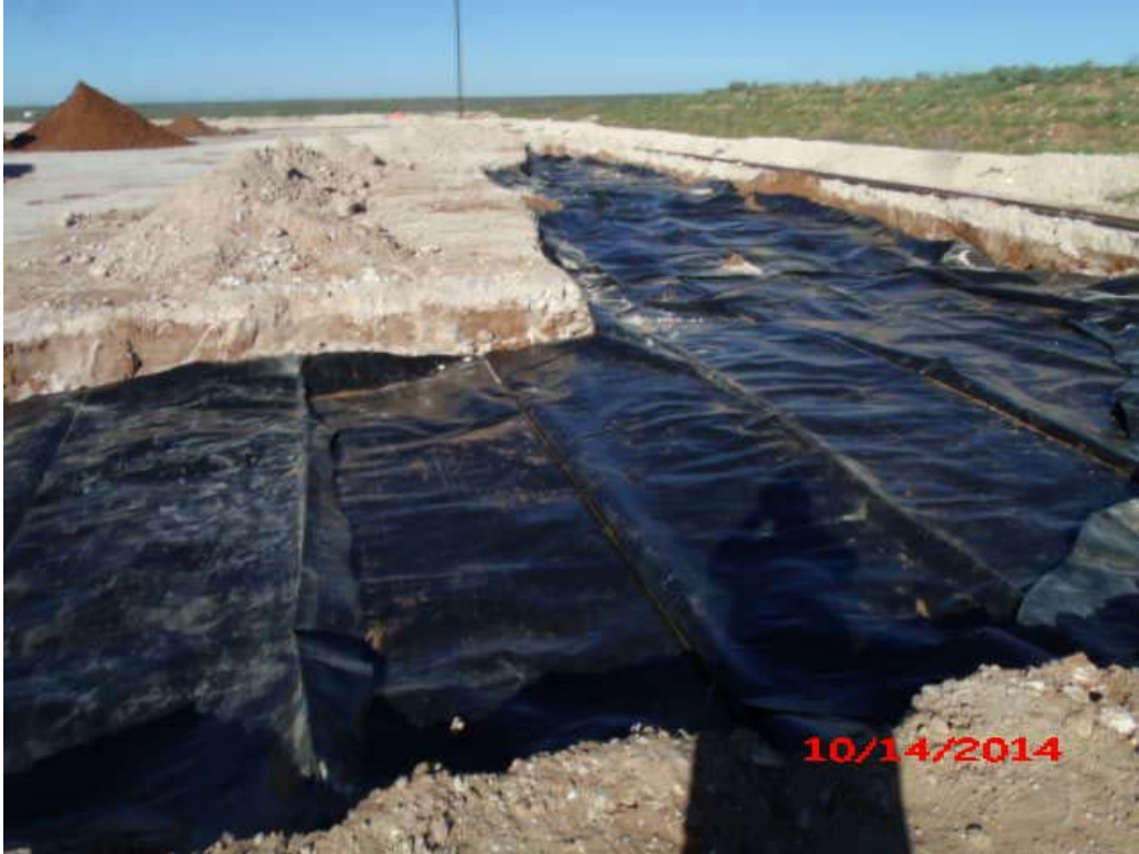
Photograph #9 – Installation of liner
