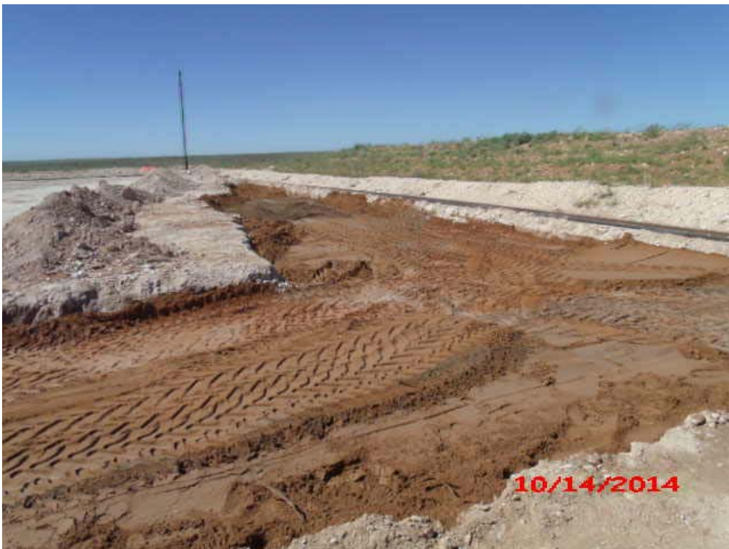
Photograph #10 – Cushion material over liner
