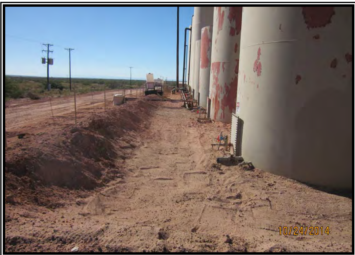
South side of the battery after backfill.
