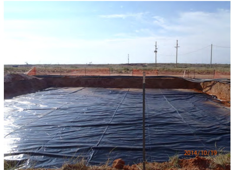
Key set of liner completed, facing south 10/19/14
