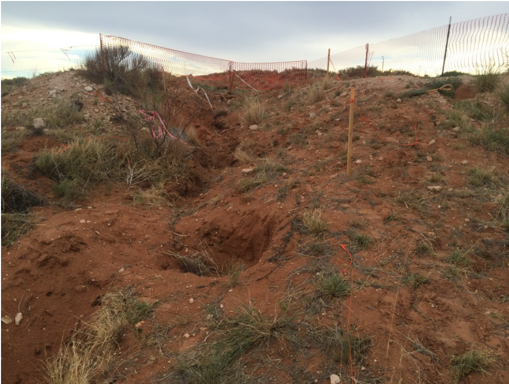
Figure 2- Erosion from pad runoff (July 16)
