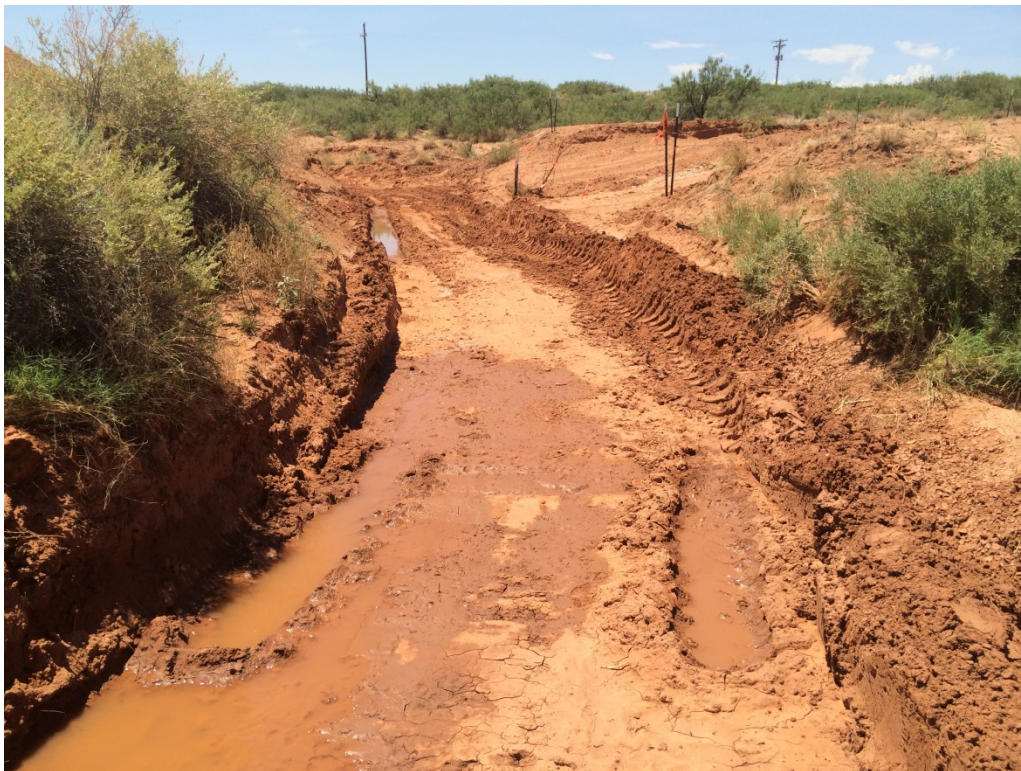
Figure 8: Nature of arroyo after removal of additional impacted material (July 30)
