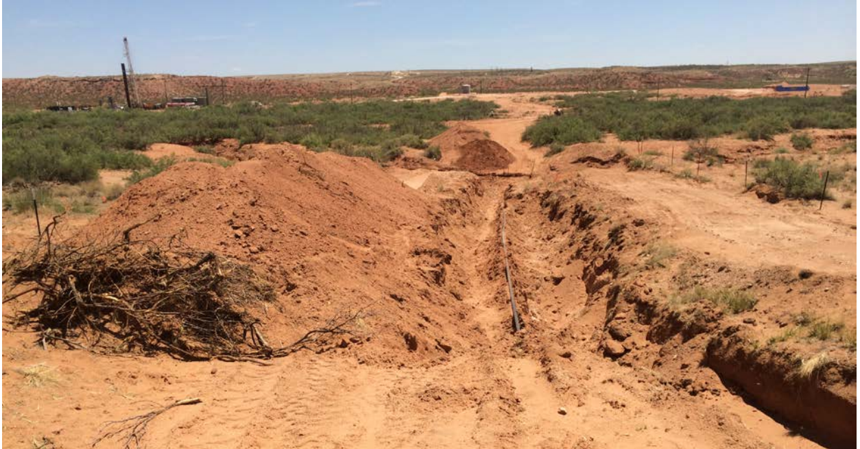
Figure 7: Nature of excavation after removal of additional impacted material (July 30). Stockpile of clean fill is left of excavation.
