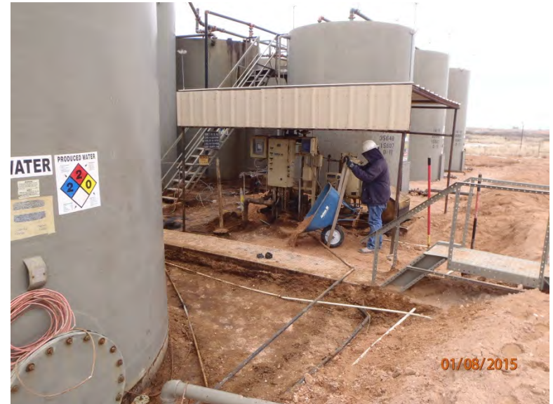
Backfilling battery, facing northwest
