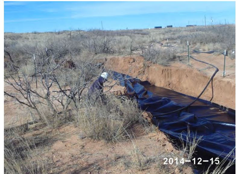
Installing liner, facing northwest 12/15/14
