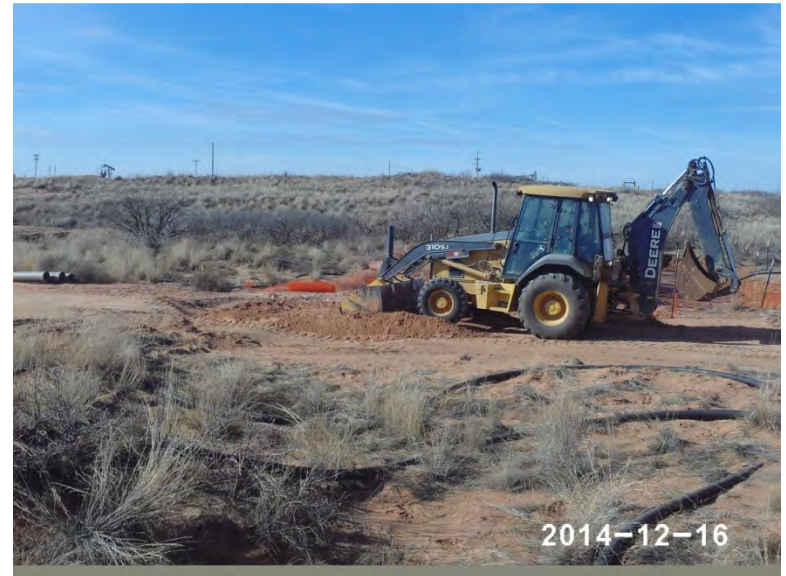
Backfilling scrape in road, facing west 12/16/14
