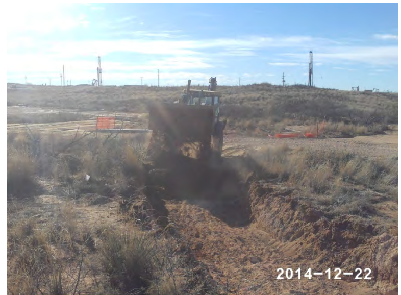
Backfilling 2 ft excavation, facing west 12/22/14
