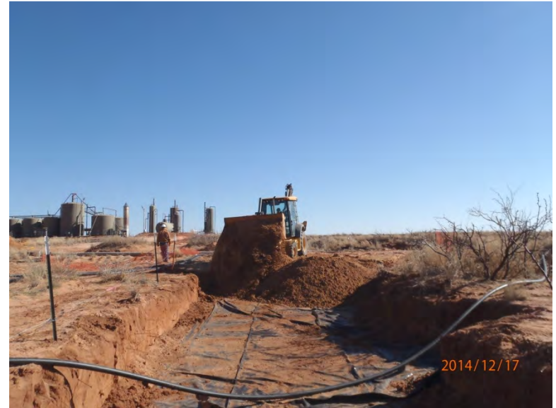
Backfilling over liner, facing east 12/17/14
