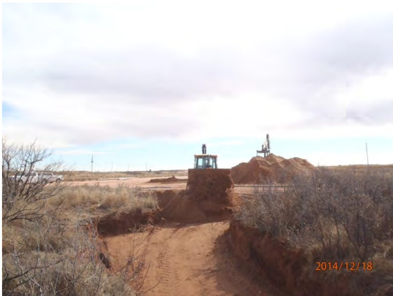
Backfilling 3 ft excavation, facing south 12/18/14
