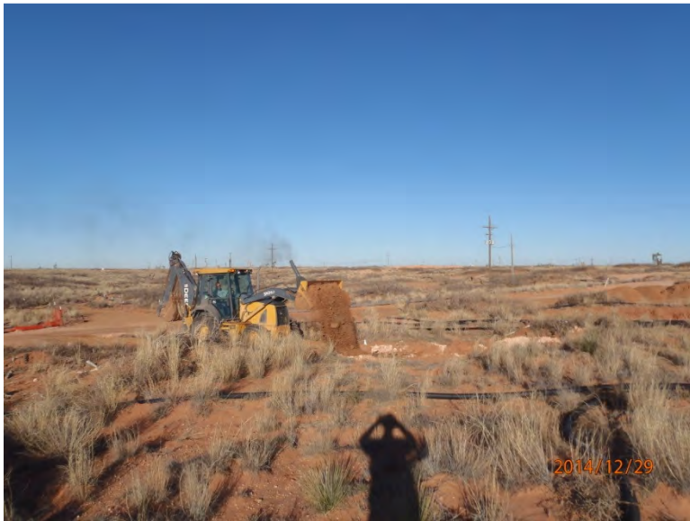
Backfilling 1.5 ft excavation, facing northwest 12/29/14
