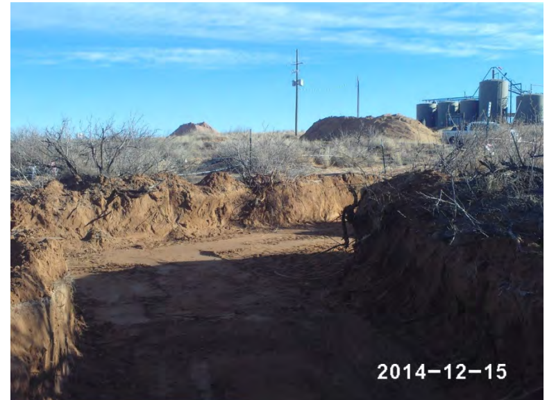
4 ft excavation completed, facing northeast 12/15/14
