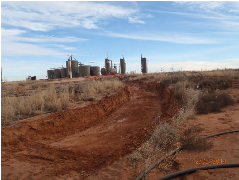
2 ft excavation completed, facing northeast 12/2/13
