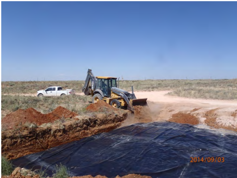
Backfilling the key set trench, facing northwest 9/3/14
