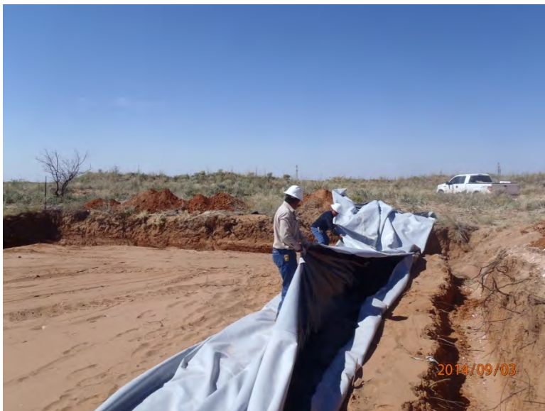
Installing 20-mil poly liner, facing west 9/3/14
