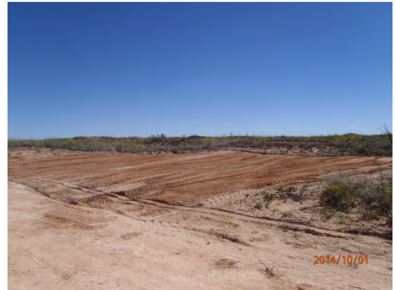
Backfilling of release area completed, facing southeast 10/1/14
