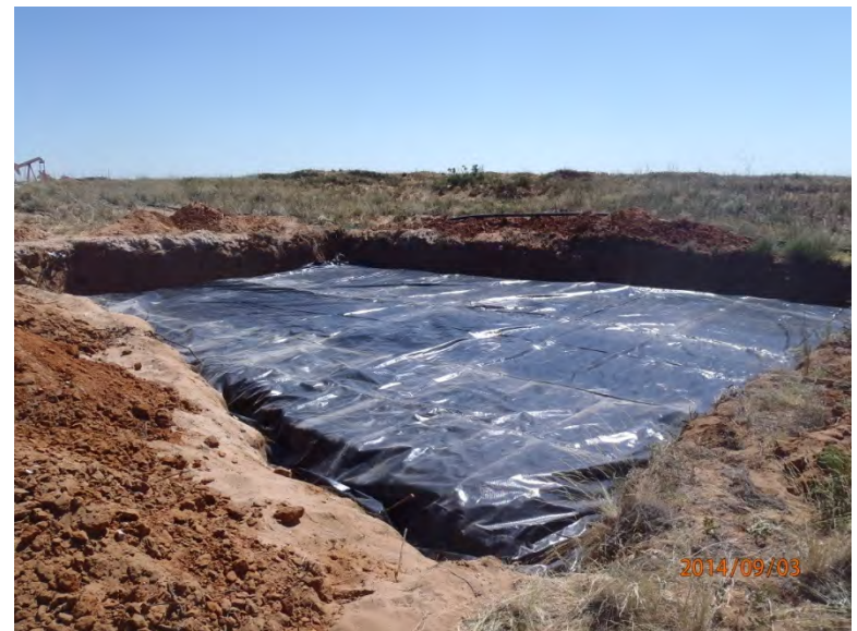
Liner installed and key set into excavation, facing southeast 9/3/14
