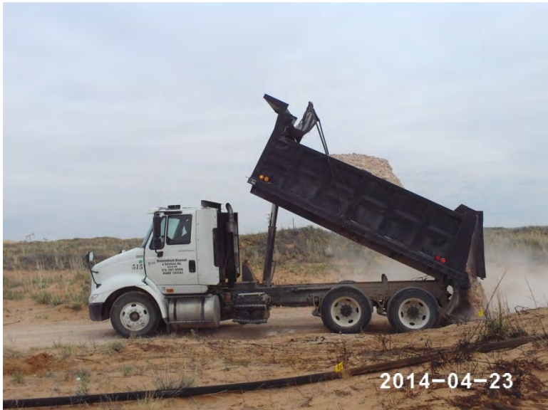
Importing caliche to build access road, facing north
