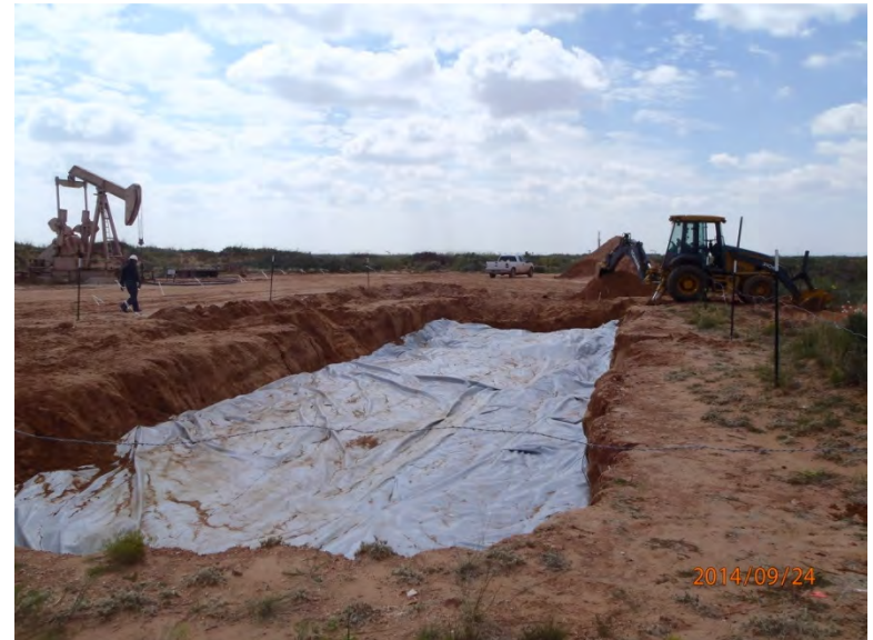
Liner installation over deep buried soil completed facing south 9/24/14
