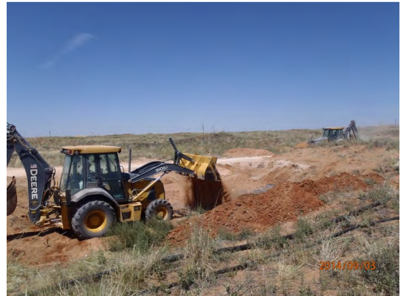
Padding liner with top soil, facing northeast 9/3/14
