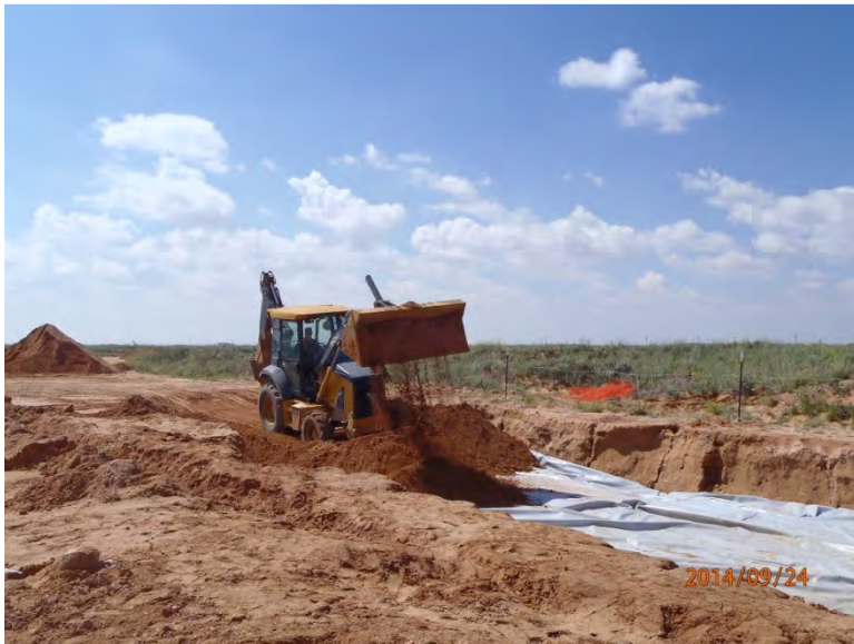
Backfilling over deep bury, facing west 9/24/14
