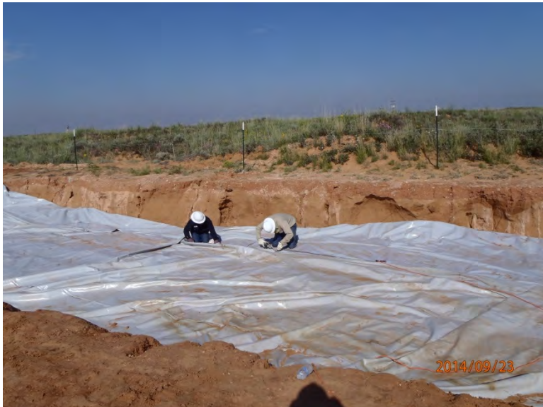
Installing liner over deep buried soil, facing west 9/23/14
