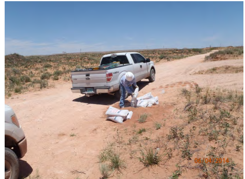
Plugging SB-3 in total with bentonite, facing northeast 6/4/14
