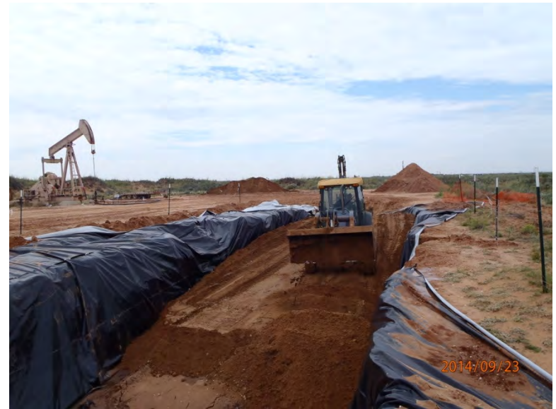
Deep burying contaminated soil, facing south 9/22/14
