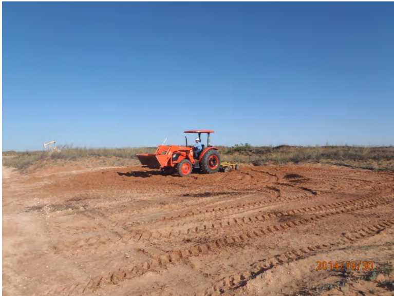
Disking in soil amendments, facing southeast 10/30/14
