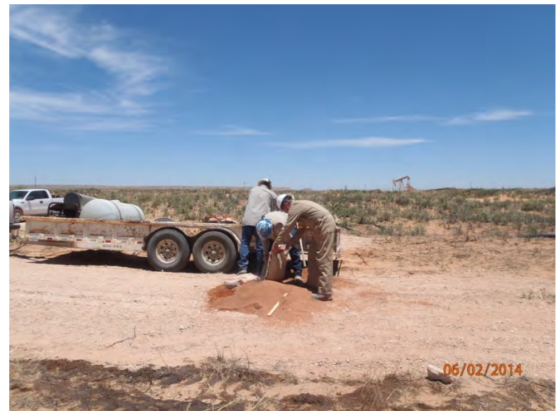
Plugging SBs in total with bentonite, facing east
