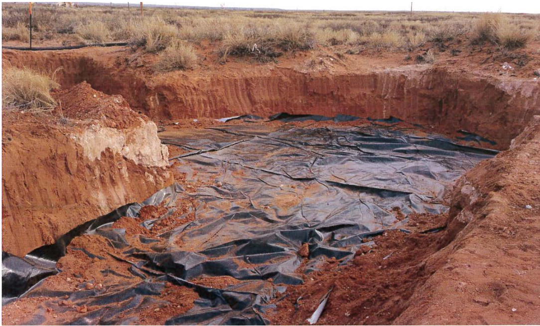
Excavated area/liner installation 12/02/2014
