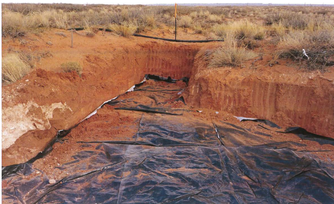
Excavated area/liner installation 12/02/2014
