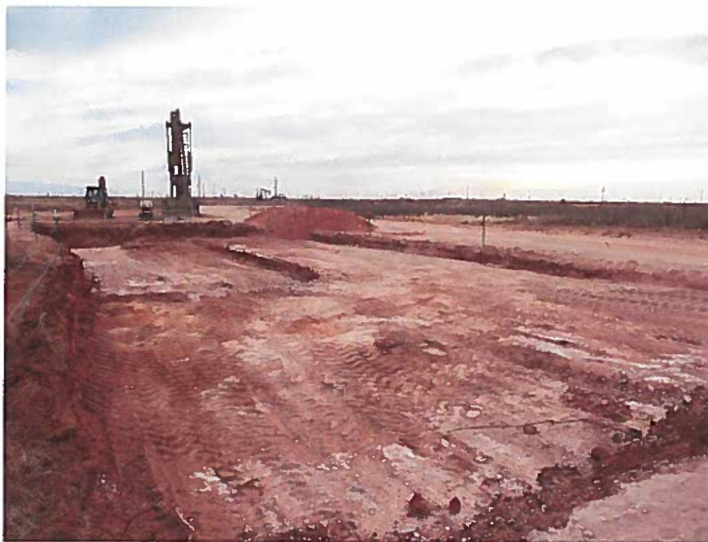
View East – Areas of AH-2, AH-3, and AH-4 Excavated
