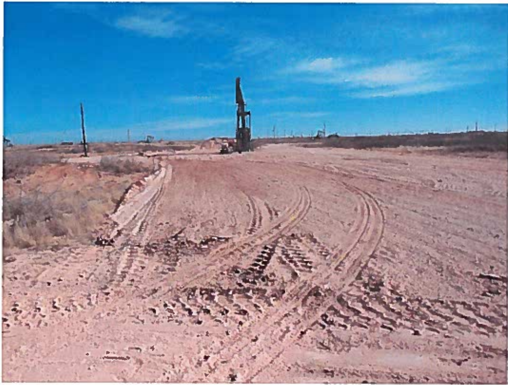
View East – Excavated Areas Backfilled
