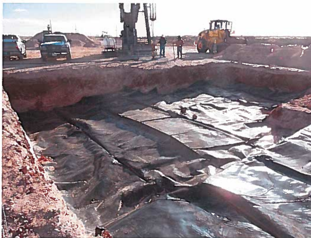
View East – Areas of AH-1 and AH-2 Lined with 40mil Plastic
