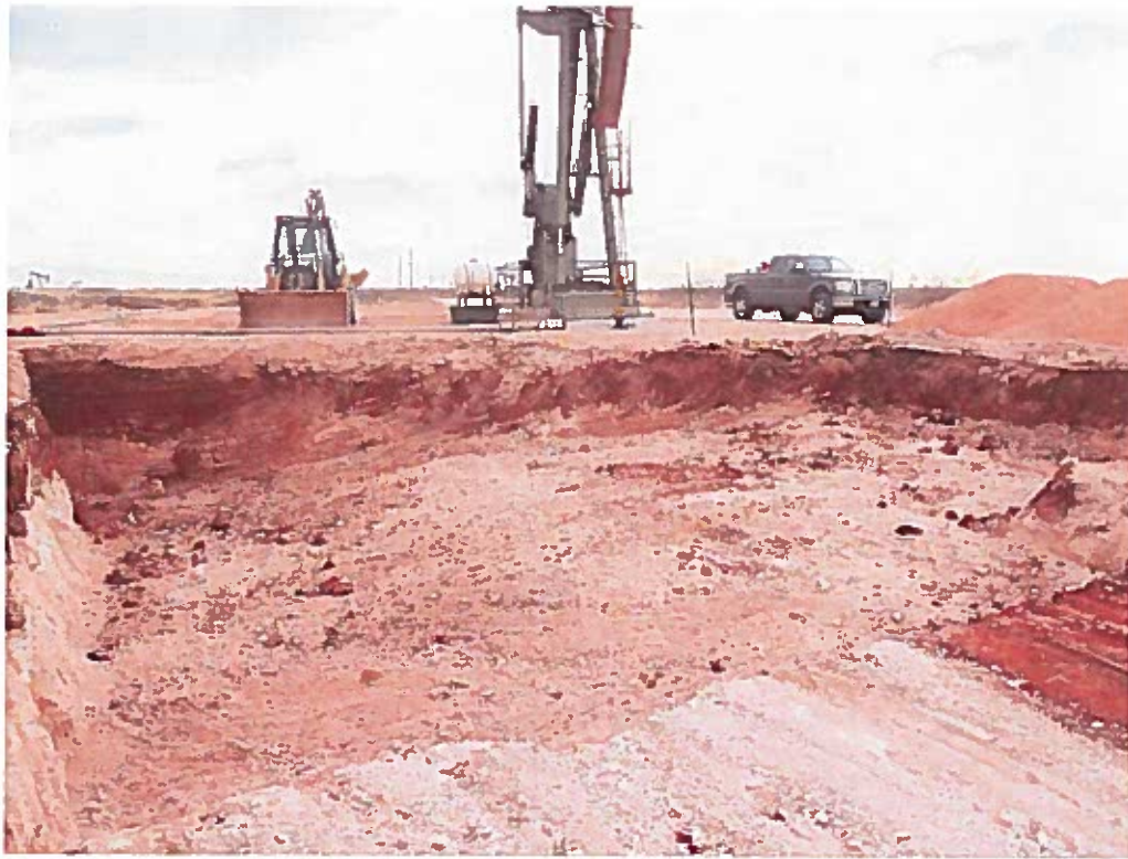
View East – Area of AH-1 at 7.0'
