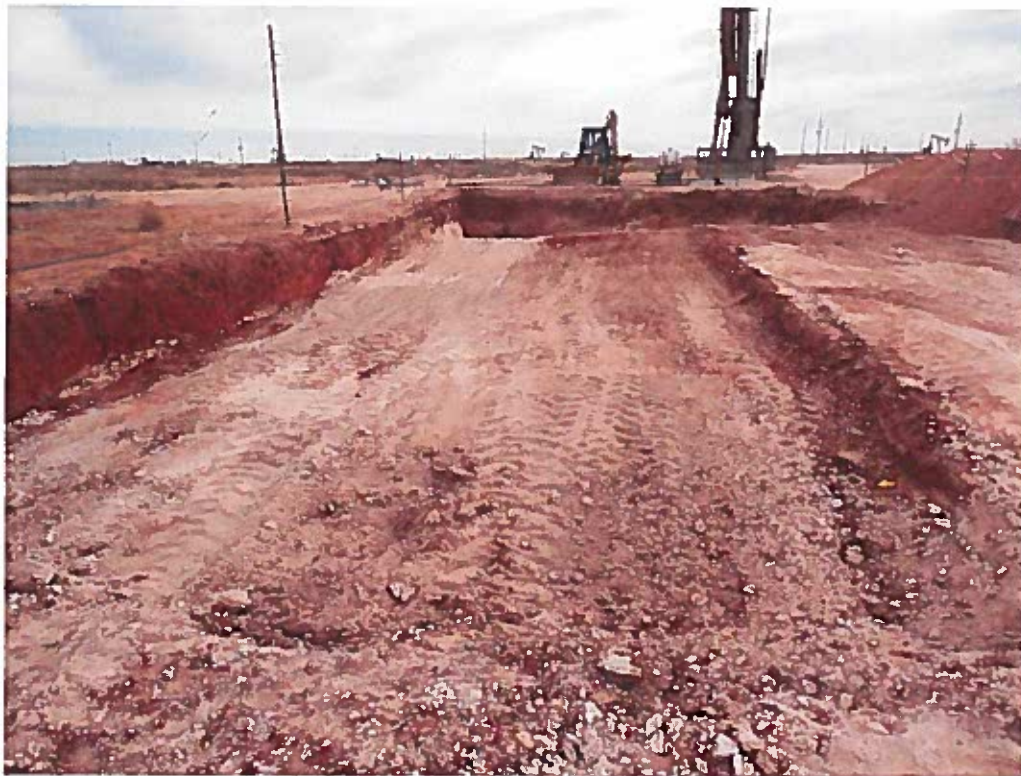
View East – Area of AH-2 at 3.0'
