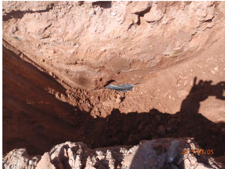
Facility liner discovered in Vertical 2
