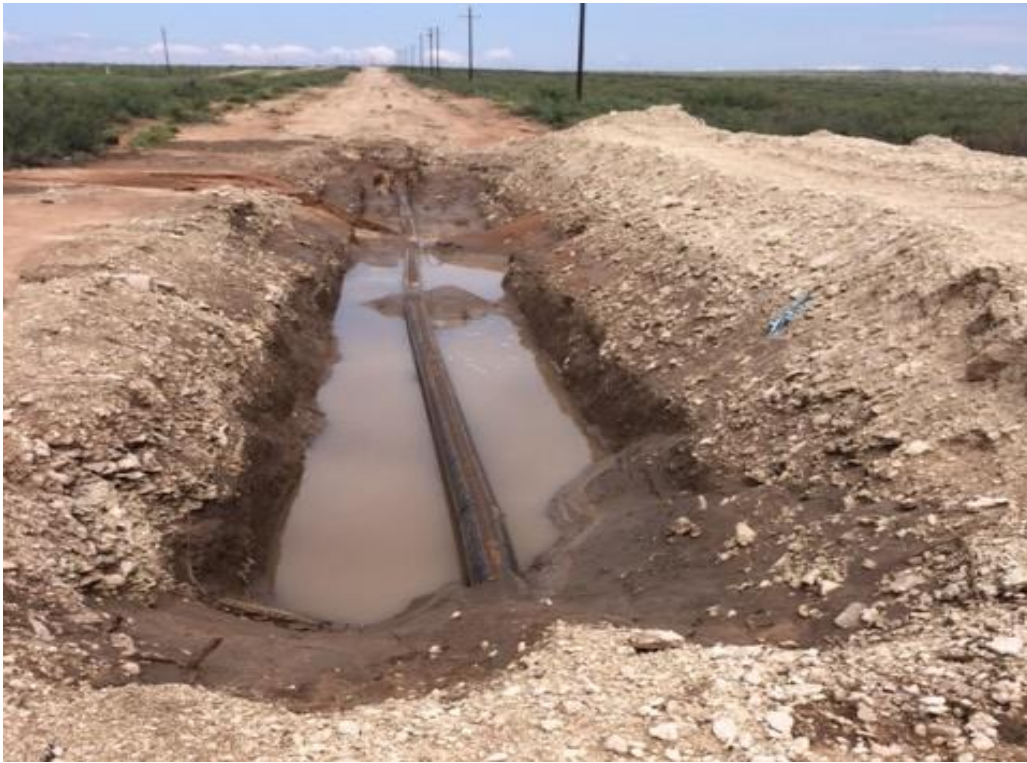
South Loop 10-Inch SWD Mainline – Excavation (Following Second Rain Event)
