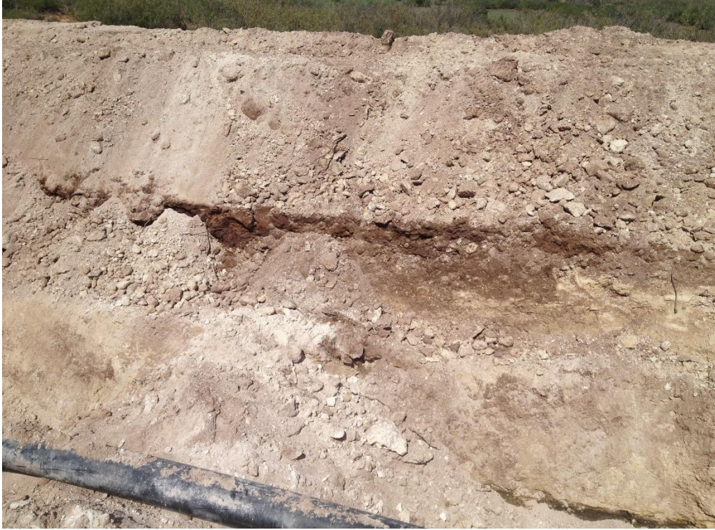
South Loop 10-Inch SWD Mainline – Staining Near Point of Release
