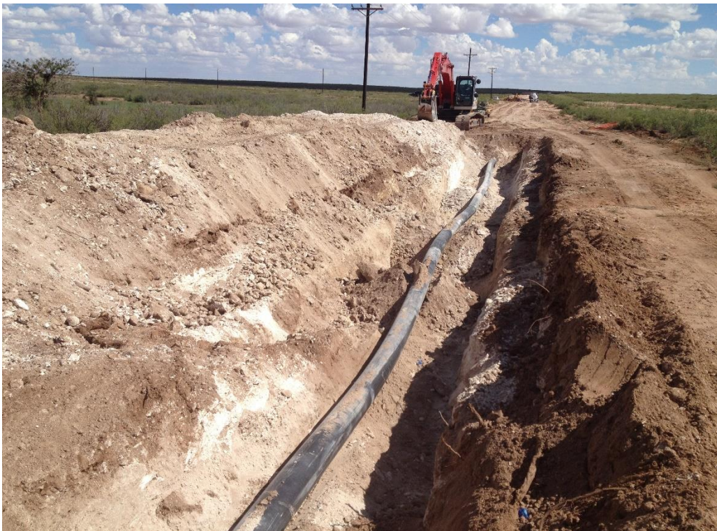
South Loop 10-Inch SWD Mainline – Excavation
