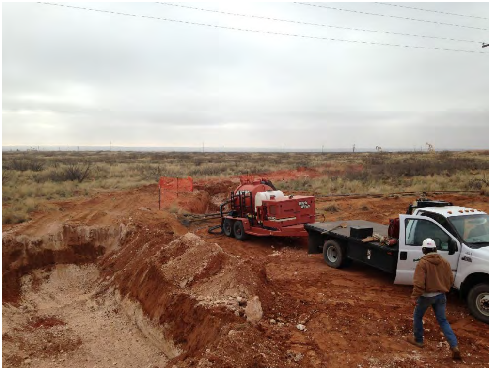
BEU-DI-9 #34H Frac Spill – Line Spotting in Excavation
