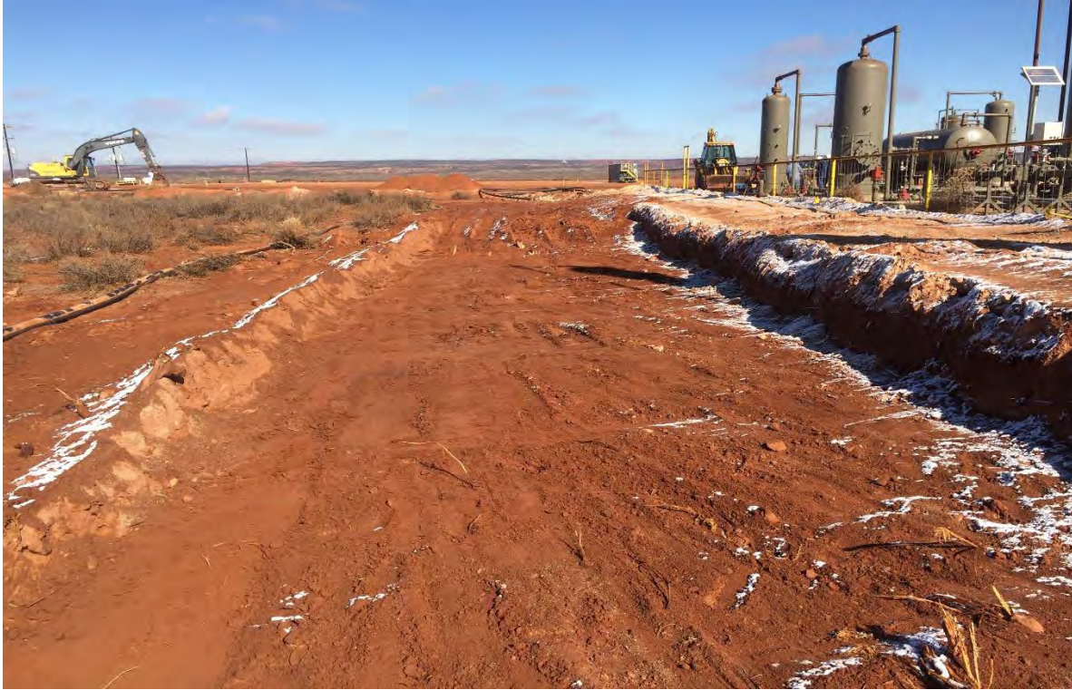
Big Eddy Unit DI-9 Tank Battery - Pasture Excavation, 11/7/2014 Release (During Backfill)
