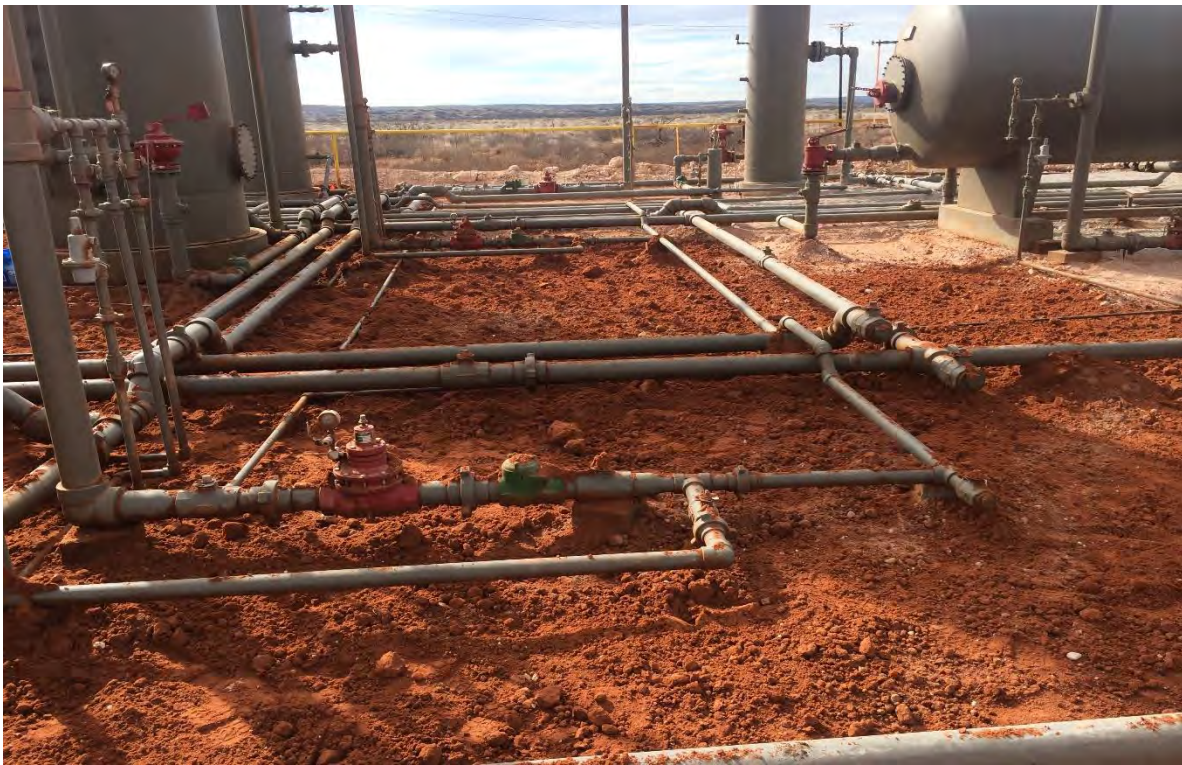
Big Eddy Unit DI-9 Tank Battery – Installation of Clay Liner, 2/9/2015 Release
