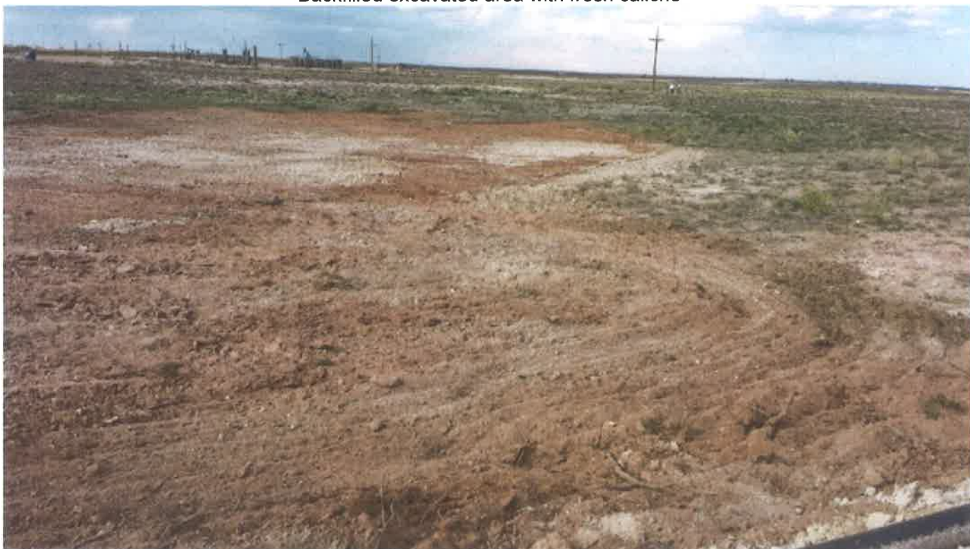
Backfilled excavated area with fresh caliche
