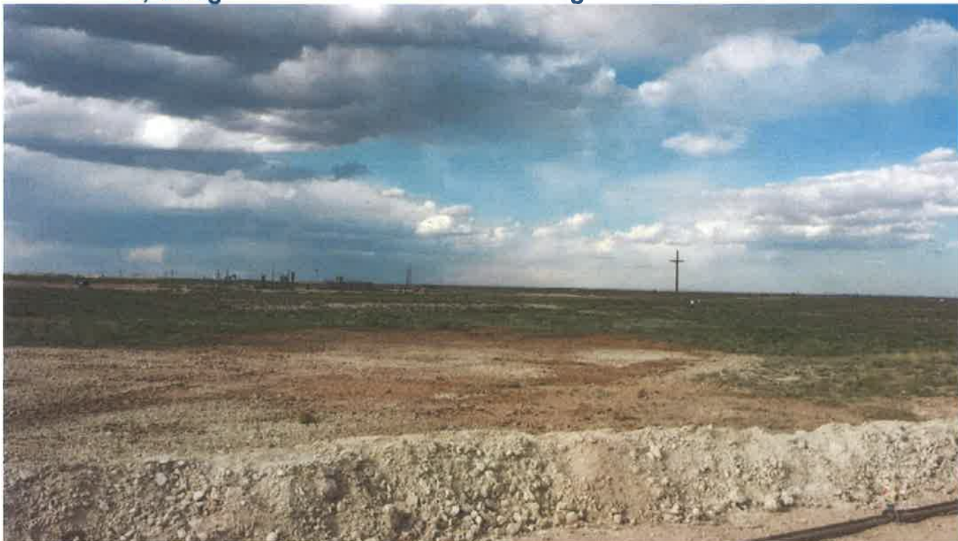
Backfilled excavated area with fresh caliche
