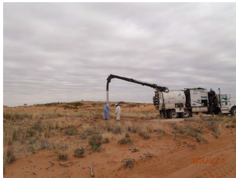
Line spot with hydrovac, facing west
