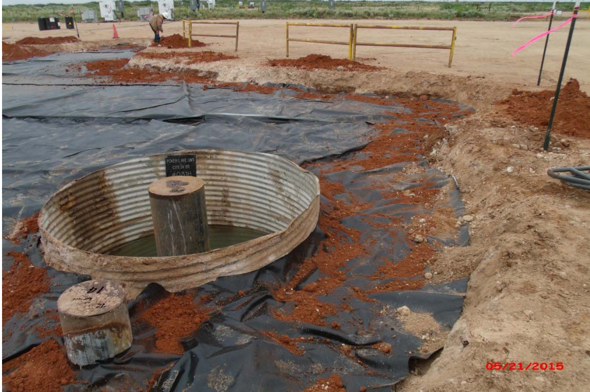
Photograph #9 – Installation of liner
