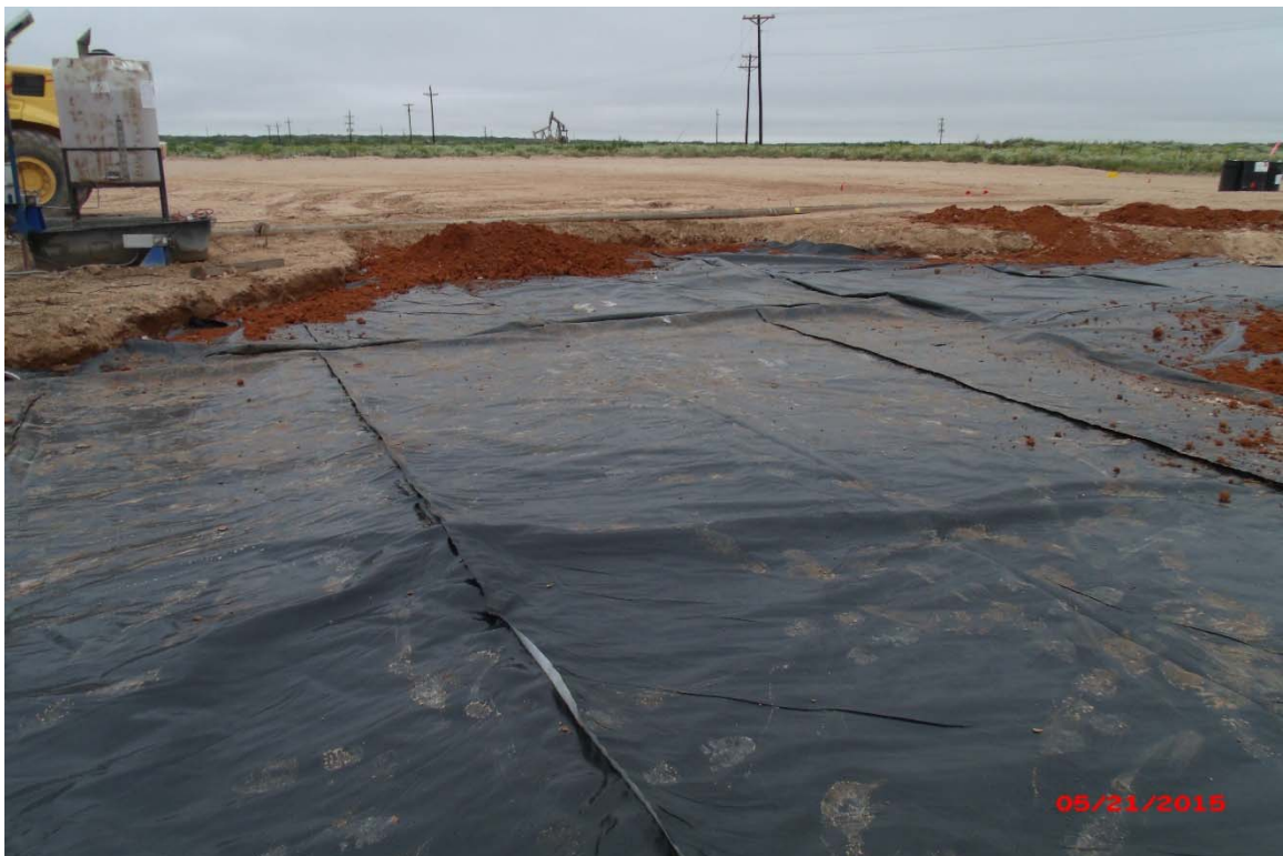
Photograph #8 – Installation of liner
