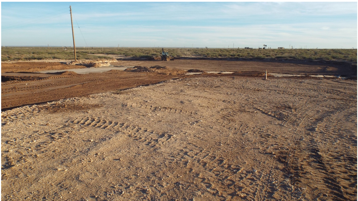
Backfilling 2 ft excavation above liner, from W pad facing SSE November 17, 2014
