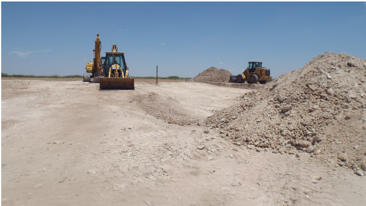
Excavating high chloride impact areas in central pad area, from SW pad facing NNE July 10, 2014
