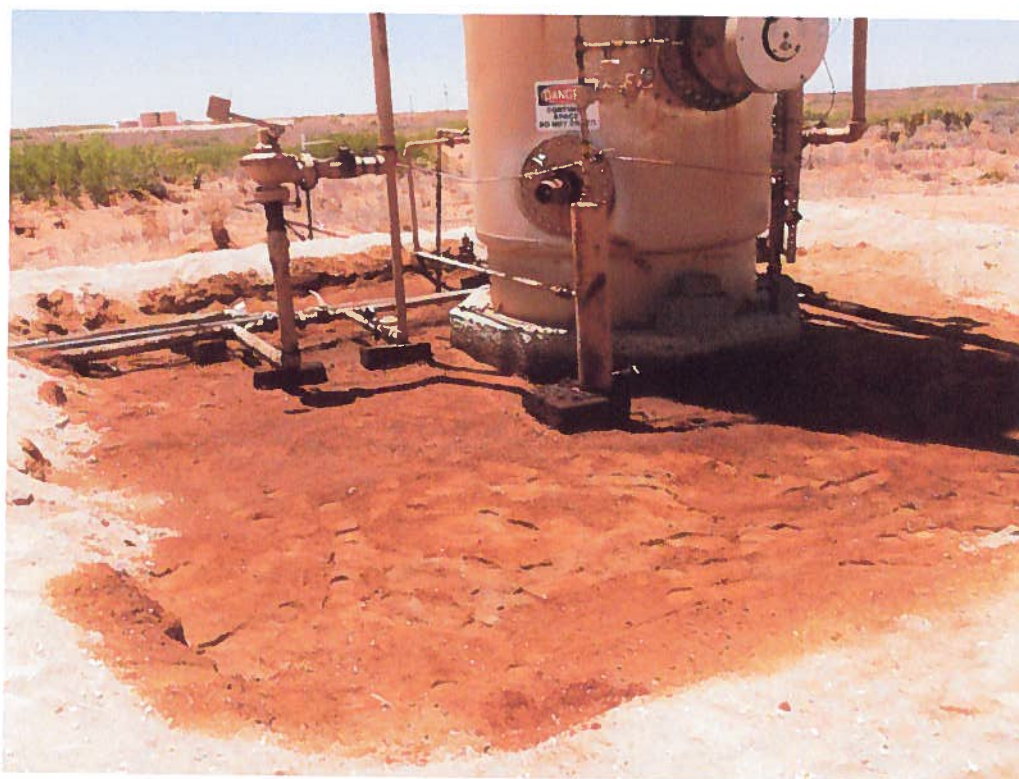
View South – Area of AH-1
