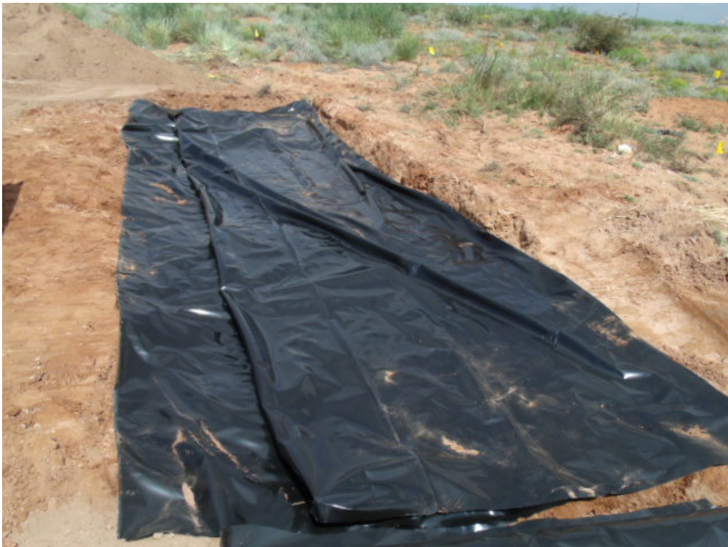
Photograph #8 – Liner installed
