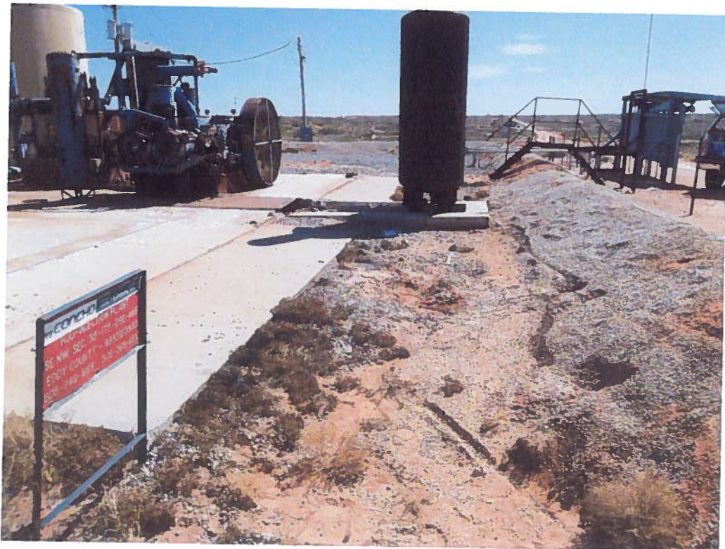
View West of AH-3
