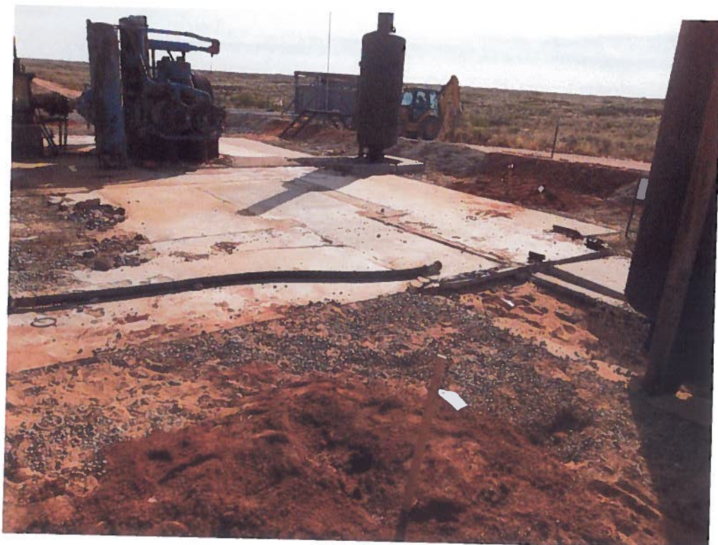
View Southeast of BH-4
