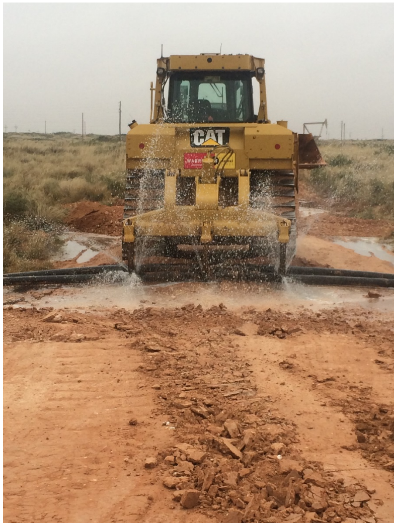
Line strike with dozer rippers in line, fluid gushing out
