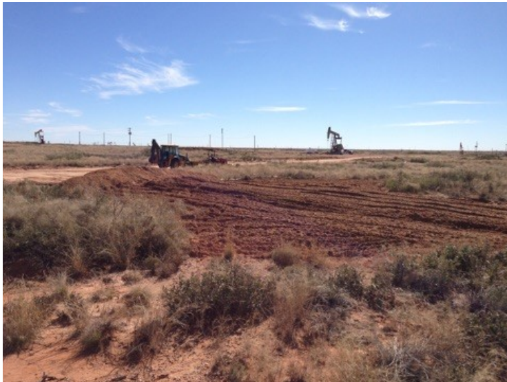
Completion of excavation area, backfilled and reseeded
