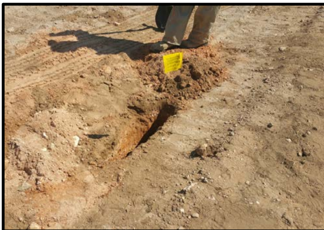
View of line located by hand digging prior to soil boring installation.
