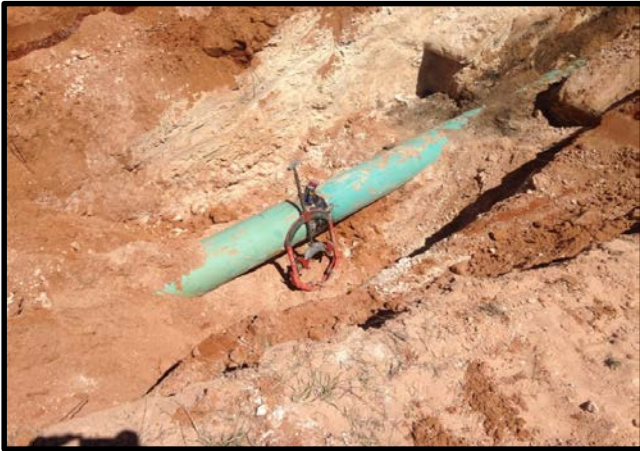
View of pipeline clamp during initial excavation activities.
