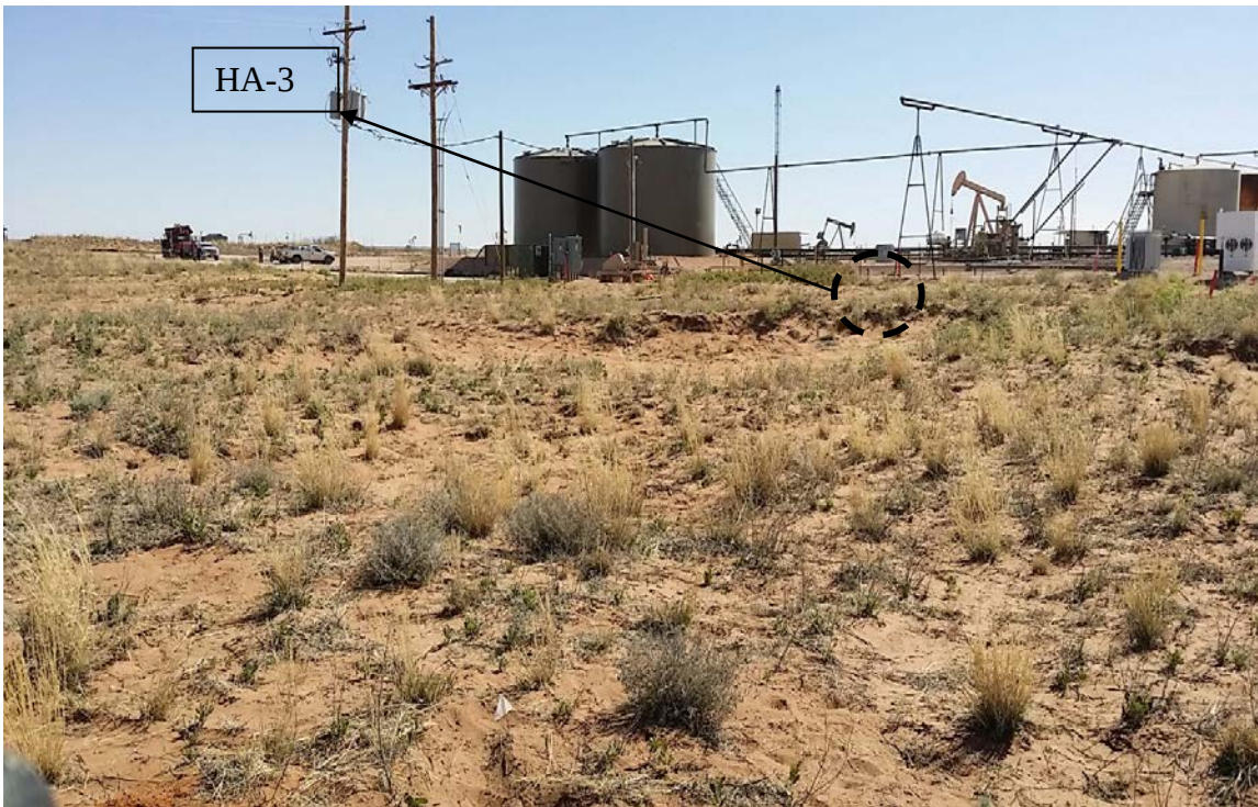
PHOTO 3: View of 2014 boring location (HA-3) and uneven sandy soil terrain facing north east
