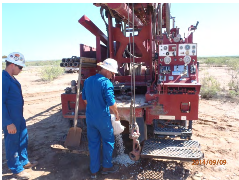
Plugging soil bores in total with bentonite, facing east
