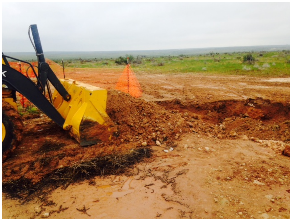
Excavating spill area behind battery in pasture
