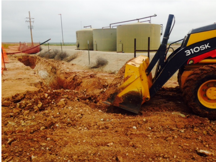
Excavating spill area behind battery in pasture
