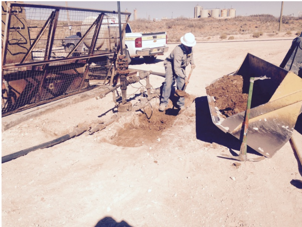
Digging out contaminated material around SP1
