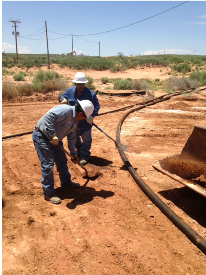
Scraping spill area around lines, wellhead
