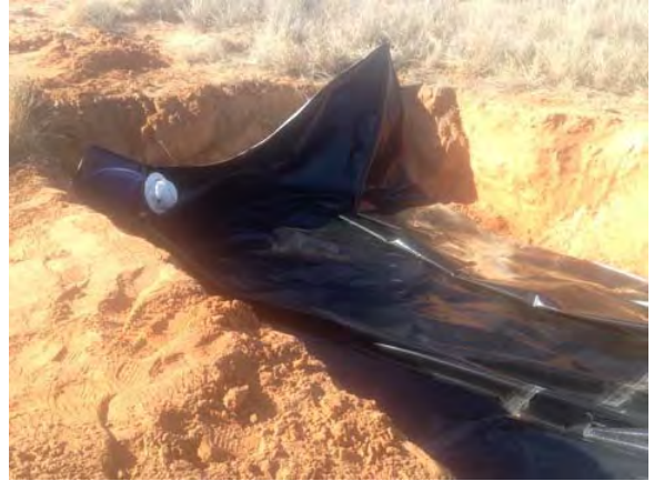
Installing 20-mil, reinforced poly liner at 4 ft bgs
