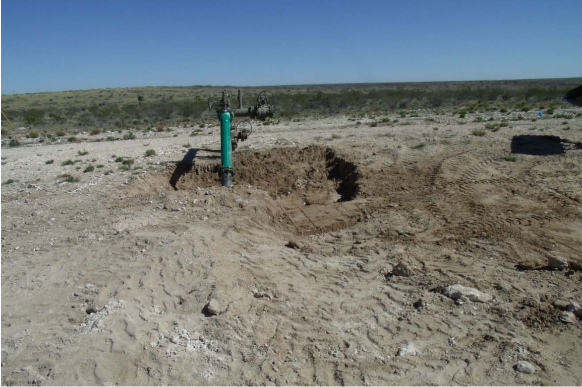
Photograph #3 – Excavated area around riser
