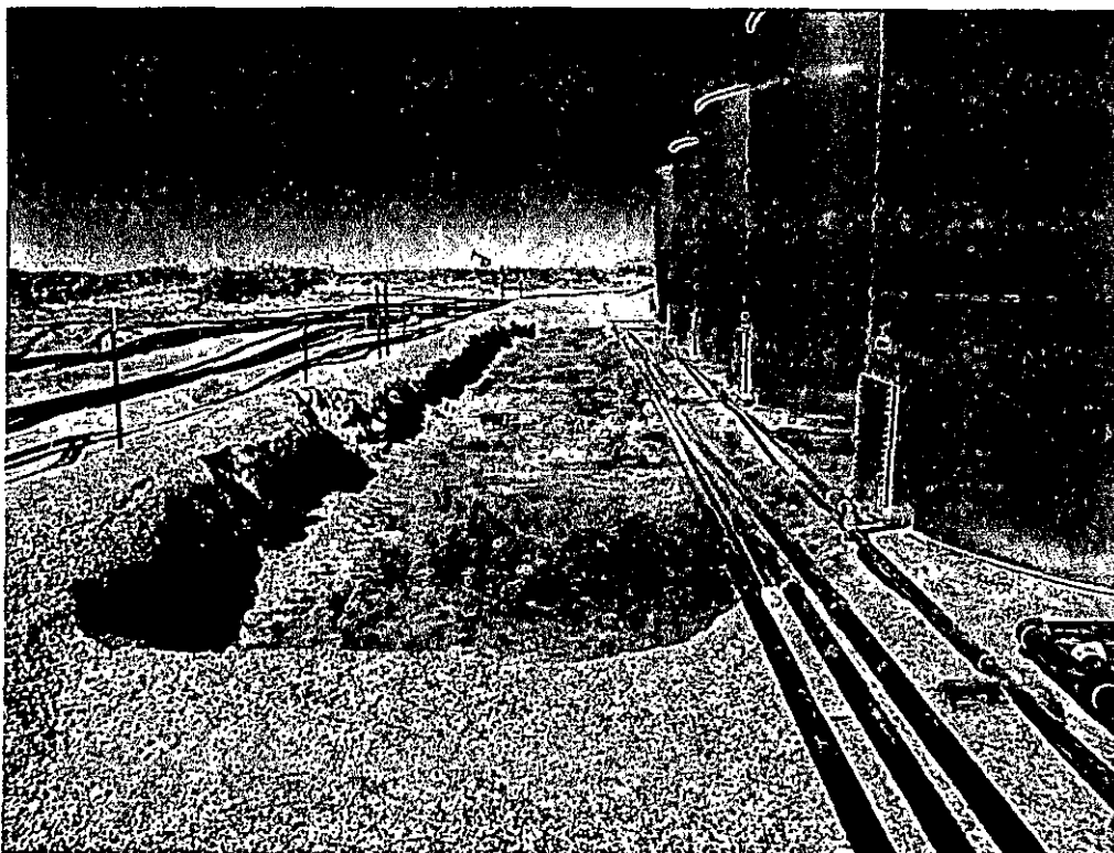
View north – Backside of tank battery near AH-1 and AH-2
