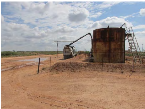
Utilizing hydrovac to collect samples 9/25/2014
