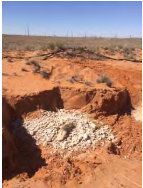
Installing river rock at the base of the 4' deep excavation
