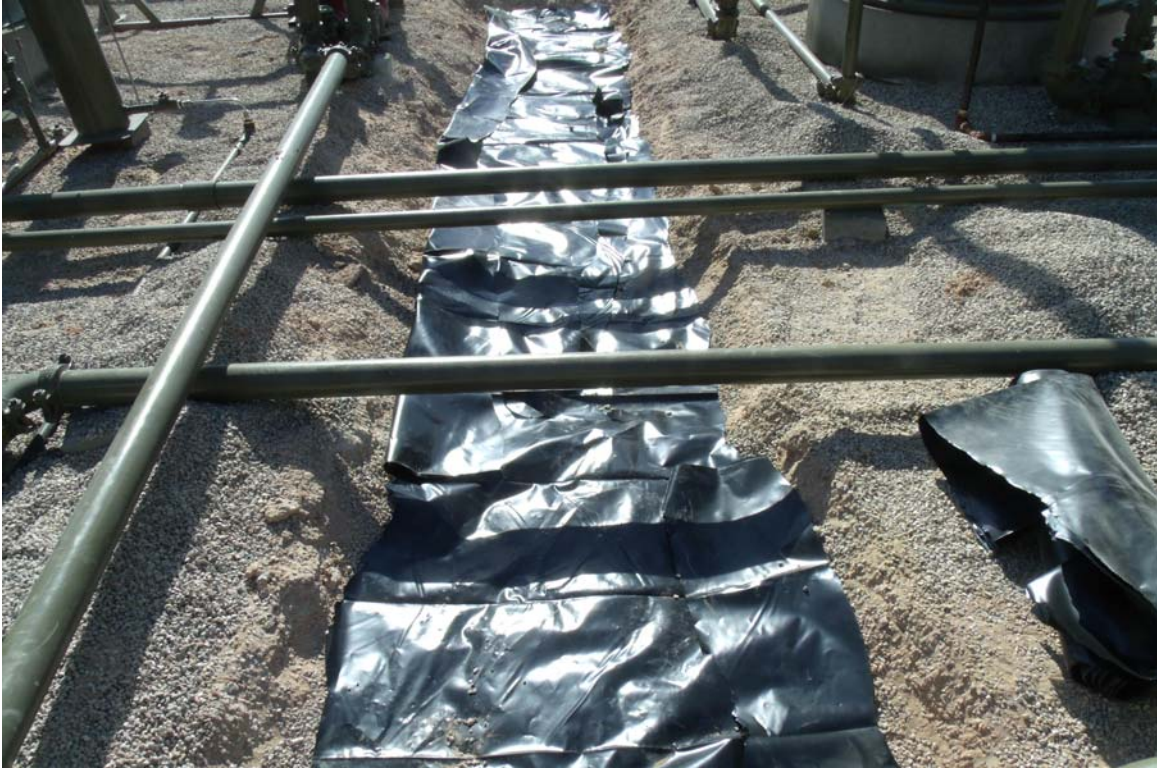
Photograph #9 – Liner installed
