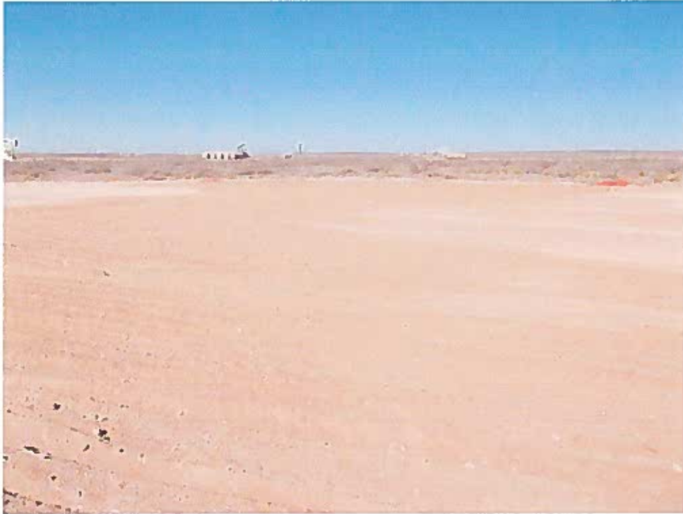
View North – Backfill
