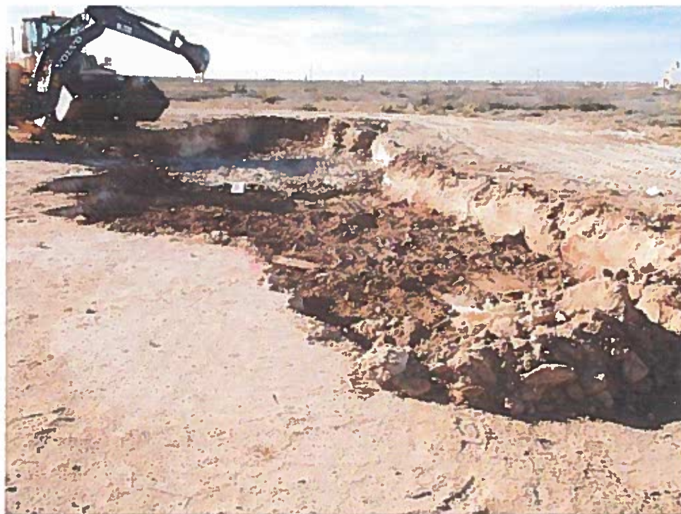
View West – Excavation of AH-5 and AH-6.
