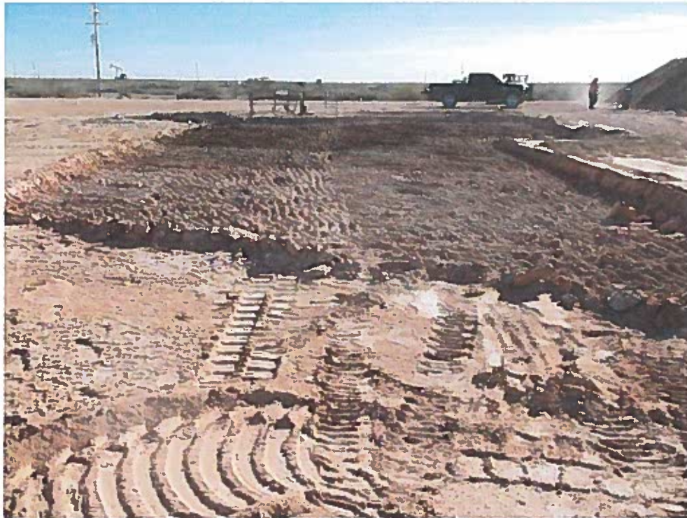
View South— Excavation of AH-4.
