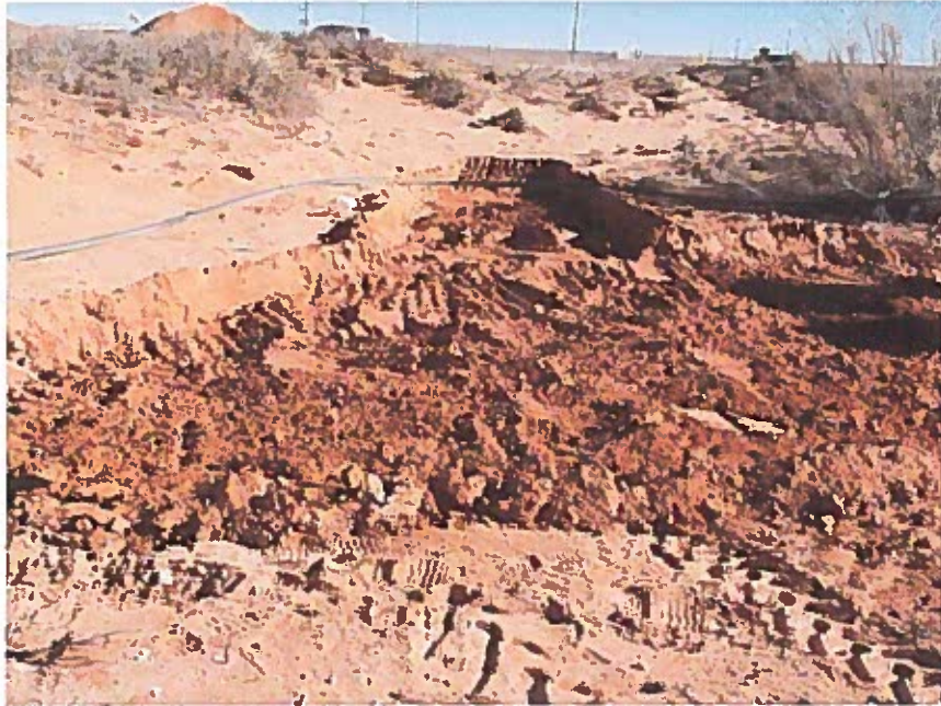
View North – Excavation of AH-1.
