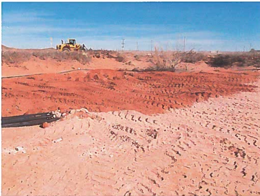
View Northeast – Backfill of AH-1 and AH-2 excavations.
