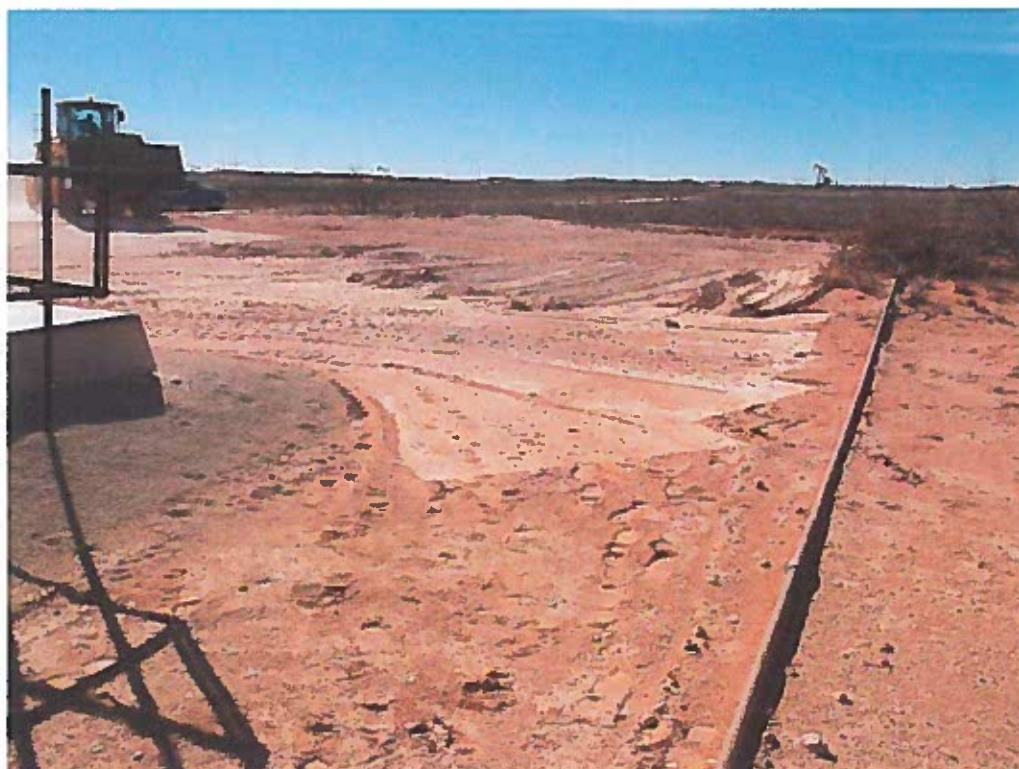
View North – Backfill of AH-5 excavation.
