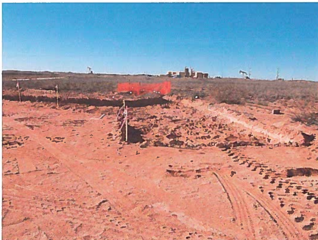
View West – Excavation of AH-5.
