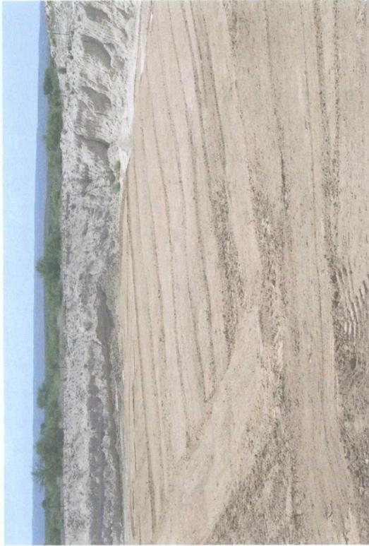
**Photo #27 – Building Bottom Crown For Liner**
