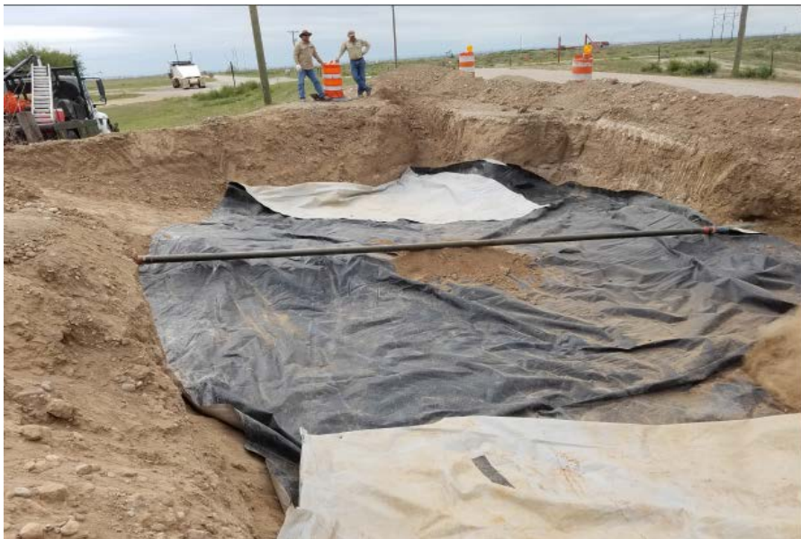
Excavated area after placing liner looking to south
