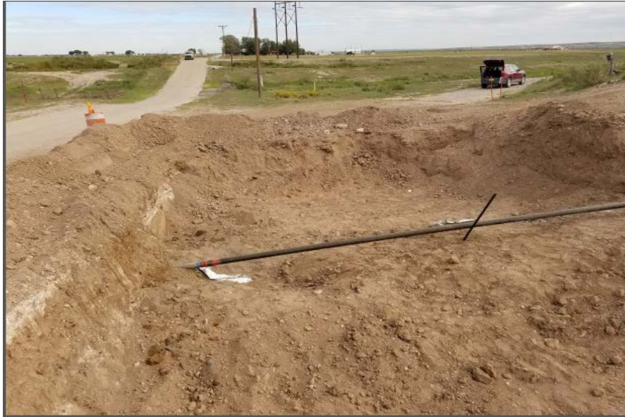
Excavated area before placing liner looking to north
