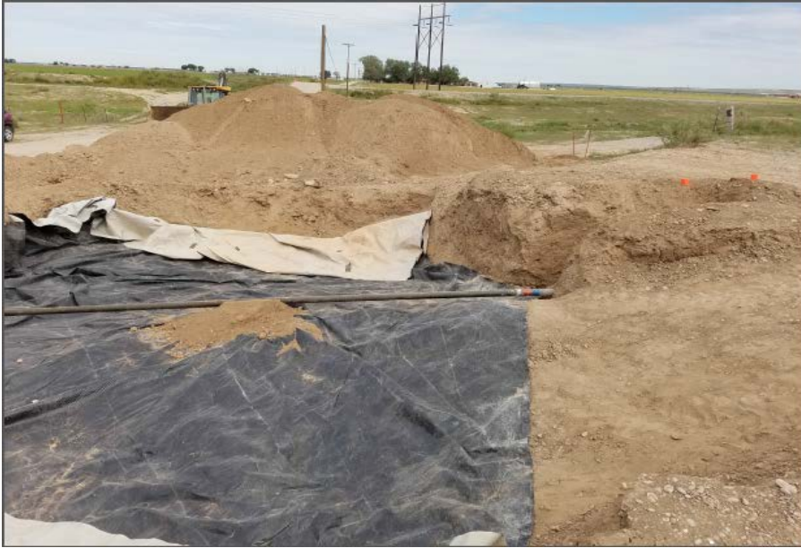
Excavated area after placing liner looking to north
