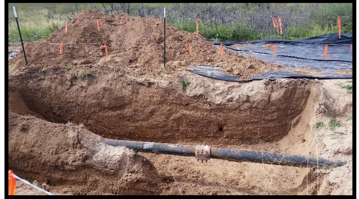
View of clamped pipeline and stockpiled soil during remediation activities, facing west.
