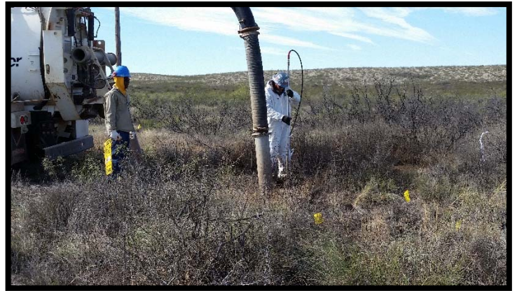
View of release point during initial hydroexcavation activities.
