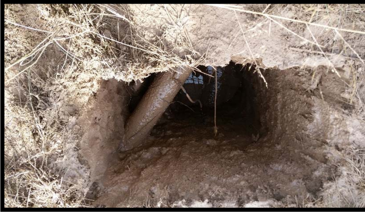
Close up view of exposed Enterprise Potash 1002 pipeline during initial hydroexcavation activities.
