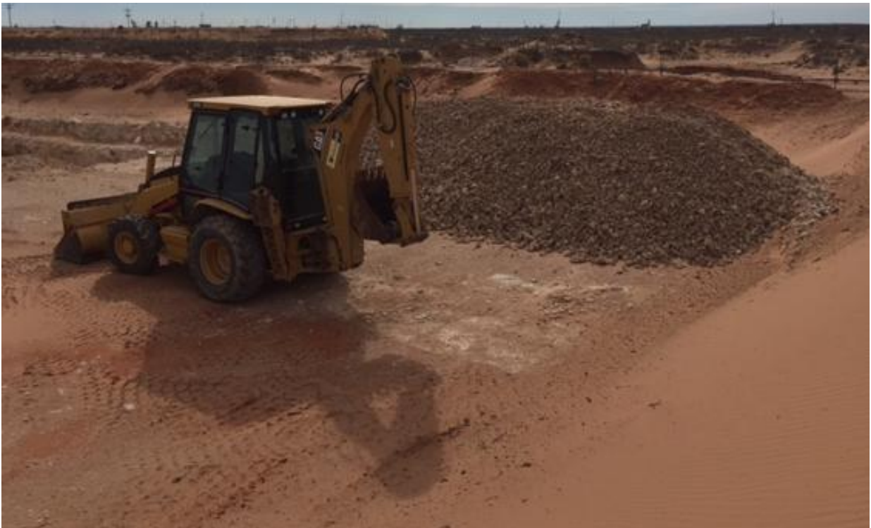
PHOTO 8: View of the remaining rock/reject stockpile proposed to be used to backfill portions of the excavated areas represented by sample points Sec. C -14 (SW. Wall), Sec. C -14 (S. Wall), Sec. D-4 and Sec. D-9, facing southeast.
