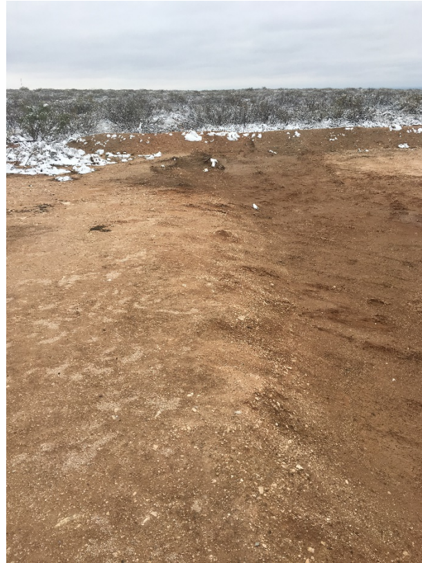
Excavation on production pad with new berms
