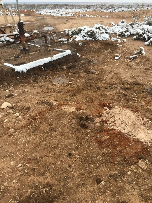
Excavation around wellhead (L4)
