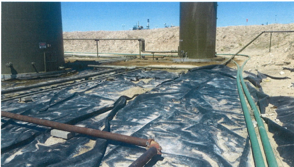
Liner East of Tanks Viewing East May 12, 2017
