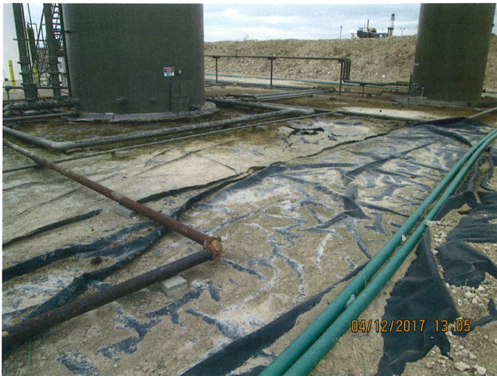
Inside Firewall after Removing Gravel Viewing Southeast
