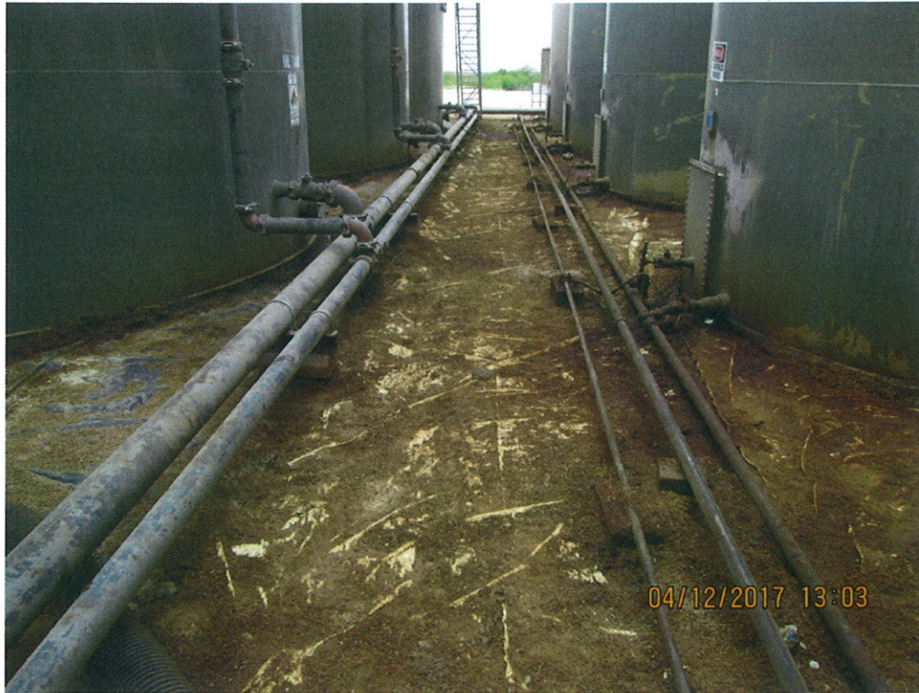
Inside Firewall after Removing Gravel Viewing West
