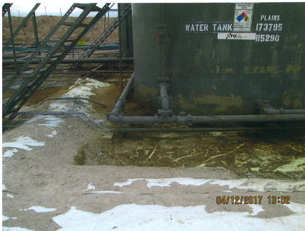
Inside Firewall after Removing Gravel Viewing South
