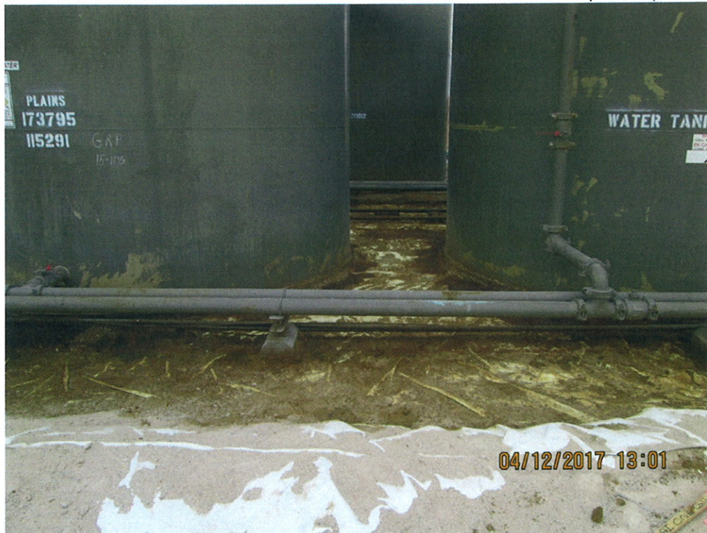
Inside Firewall after Removing Gravel Viewing South
