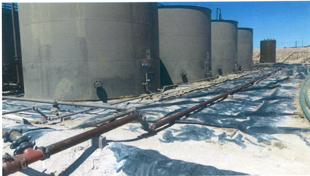
Liner South of Tanks Viewing West May 12, 2017
