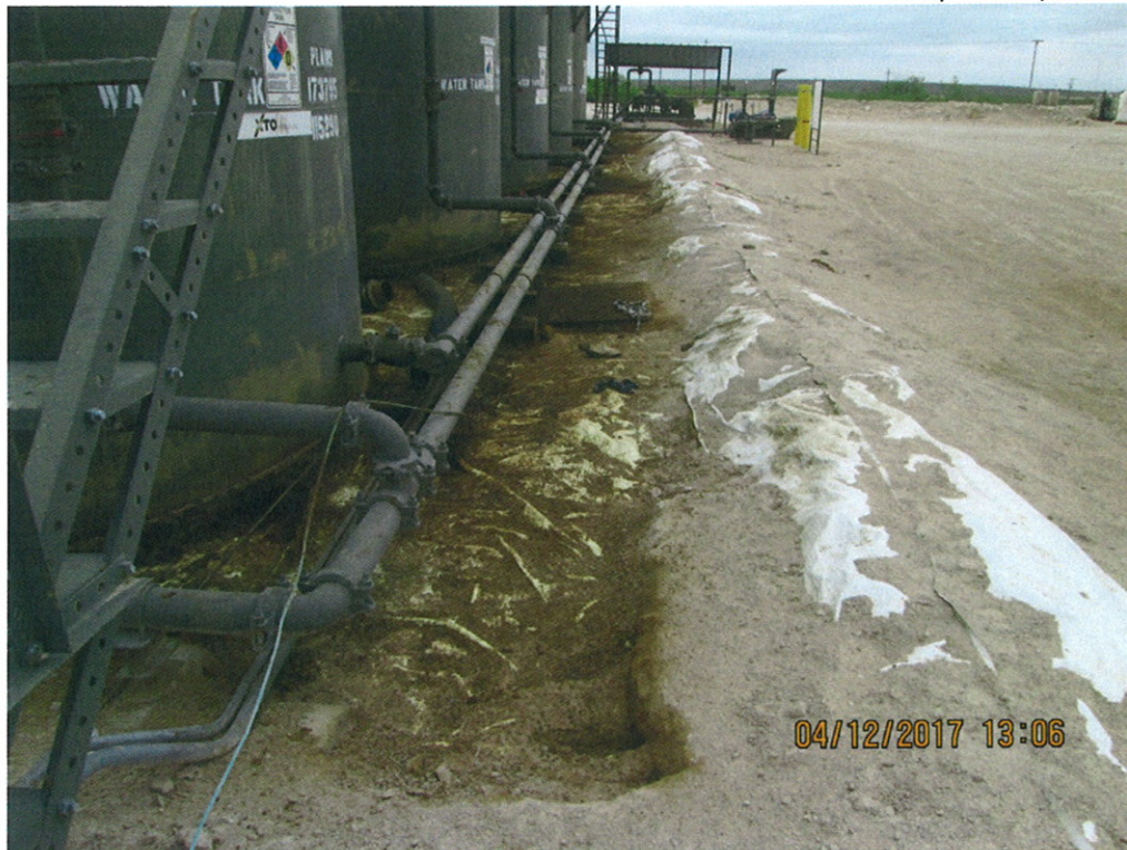
Inside Firewall after Removing Gravel Viewing West
