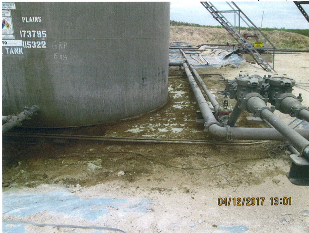
Inside Firewall after Removing Gravel Viewing South
