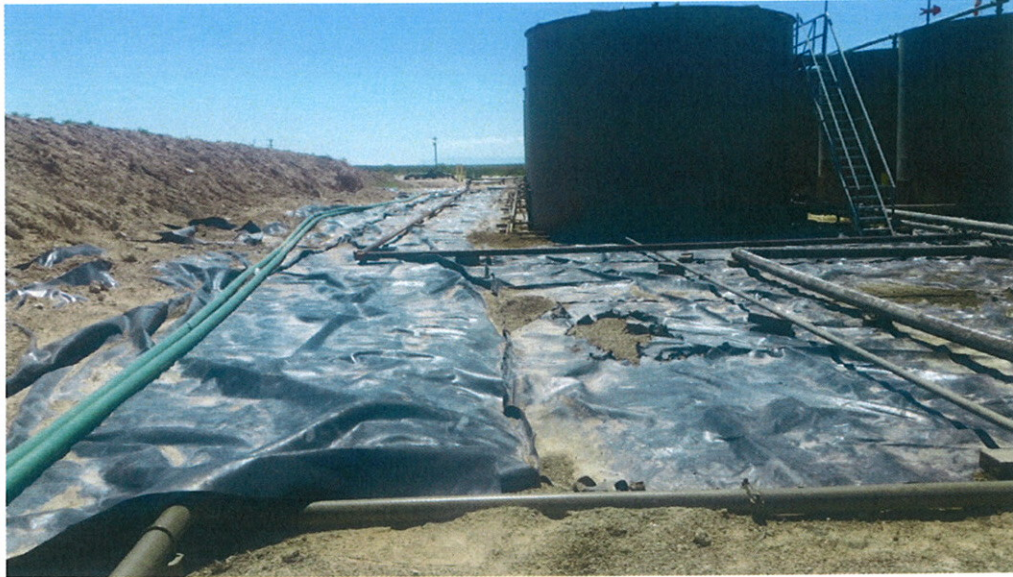
Liner East of Tanks Viewing West May 12, 2017
