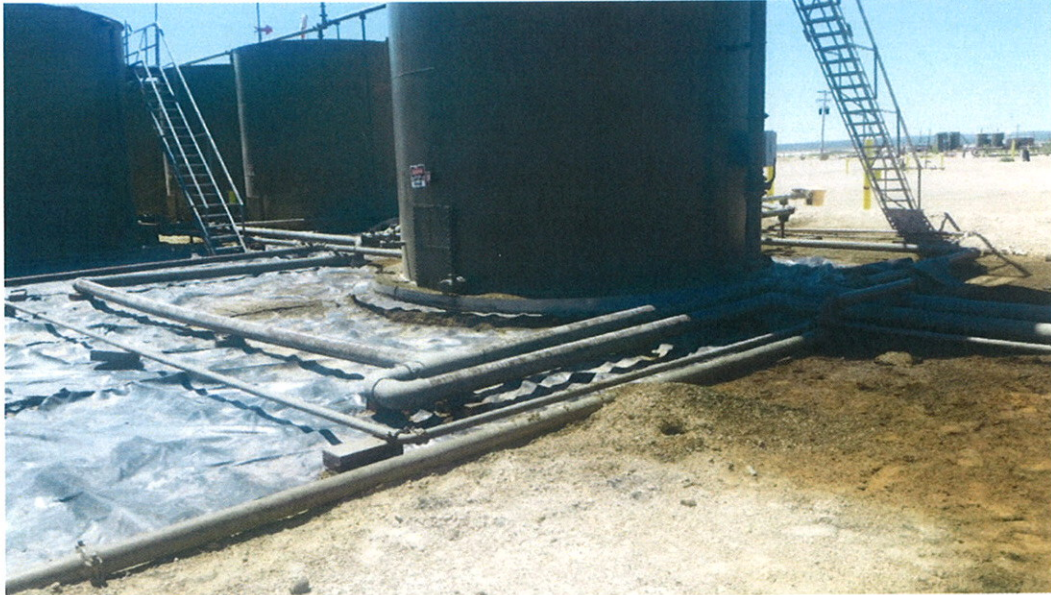
Liner East of Tanks Viewing Northwest May 12, 2017
