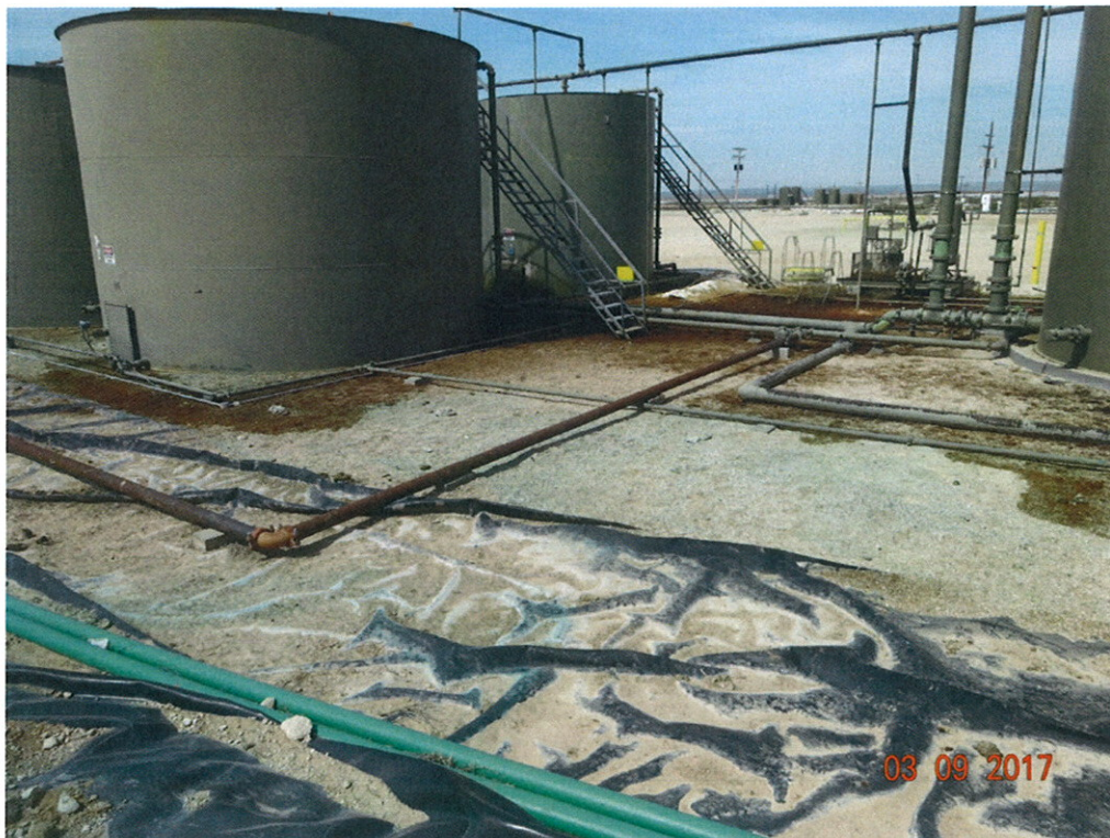
Spill Area Viewing Northwest
