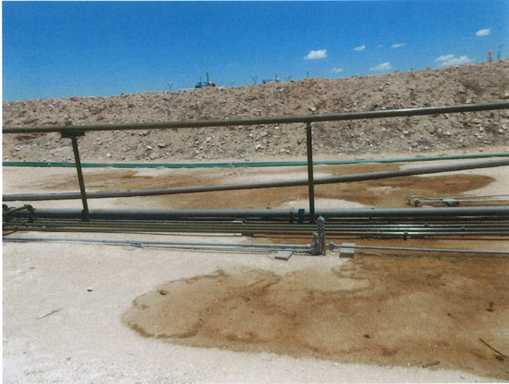
New Spill (June 14, 2017) Viewing East, June 27, 2017
