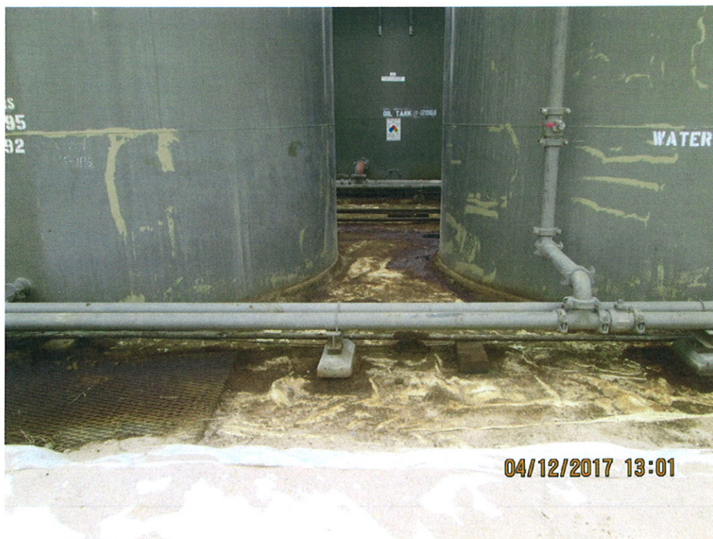
Inside Firewall after Removing Gravel Viewing South
