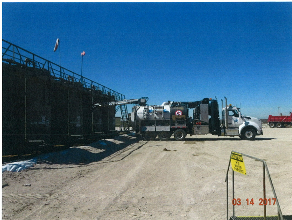
Hydrovac Truck Removing Gravel Viewing West
