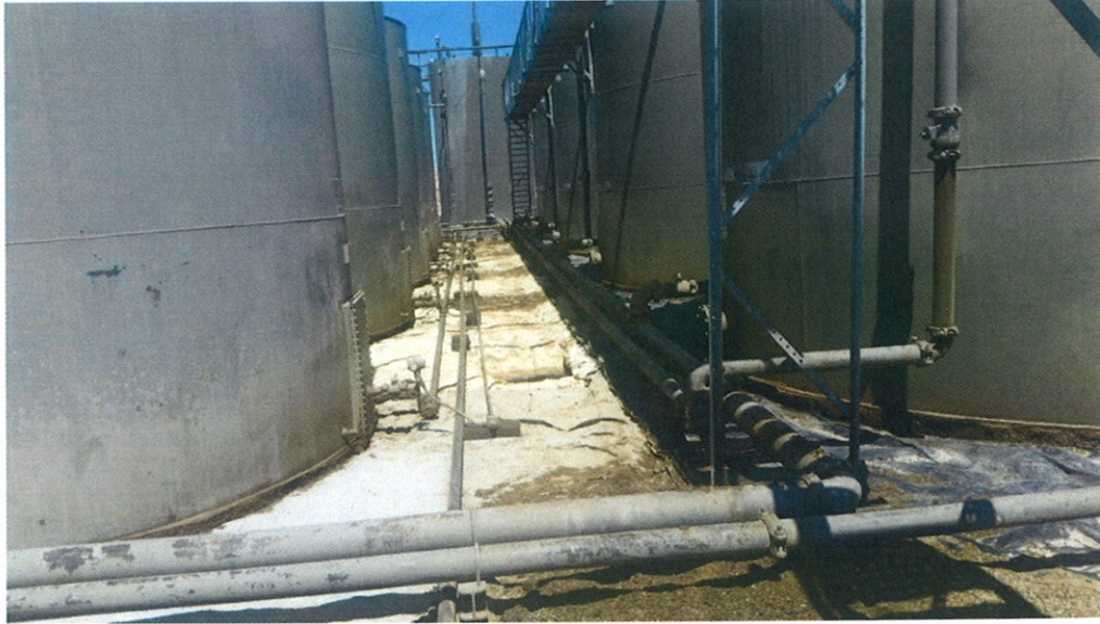
Liner inside Firewall Viewing West May 12, 2017
