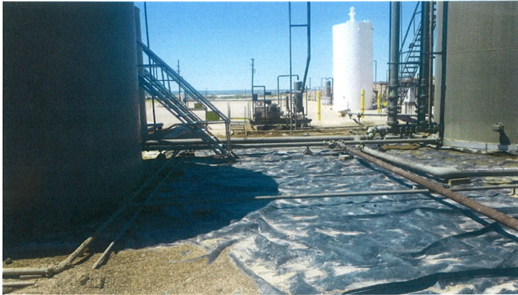
Liner East of Tanks Viewing North May 12, 2017
