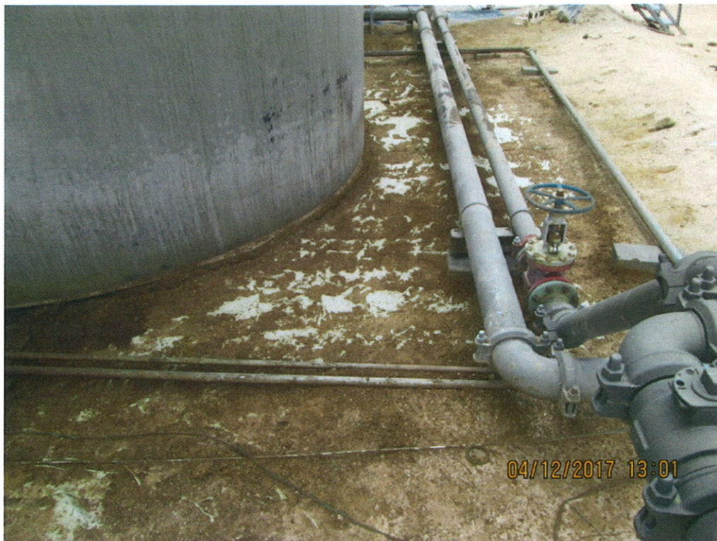
Inside Firewall after Removing Gravel Viewing West
