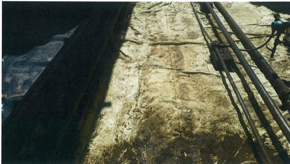
Liner inside Firewall May 12, 2017
