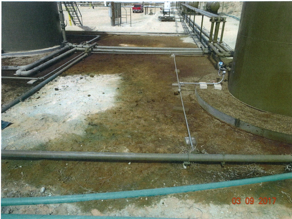
Spill Area Viewing North
