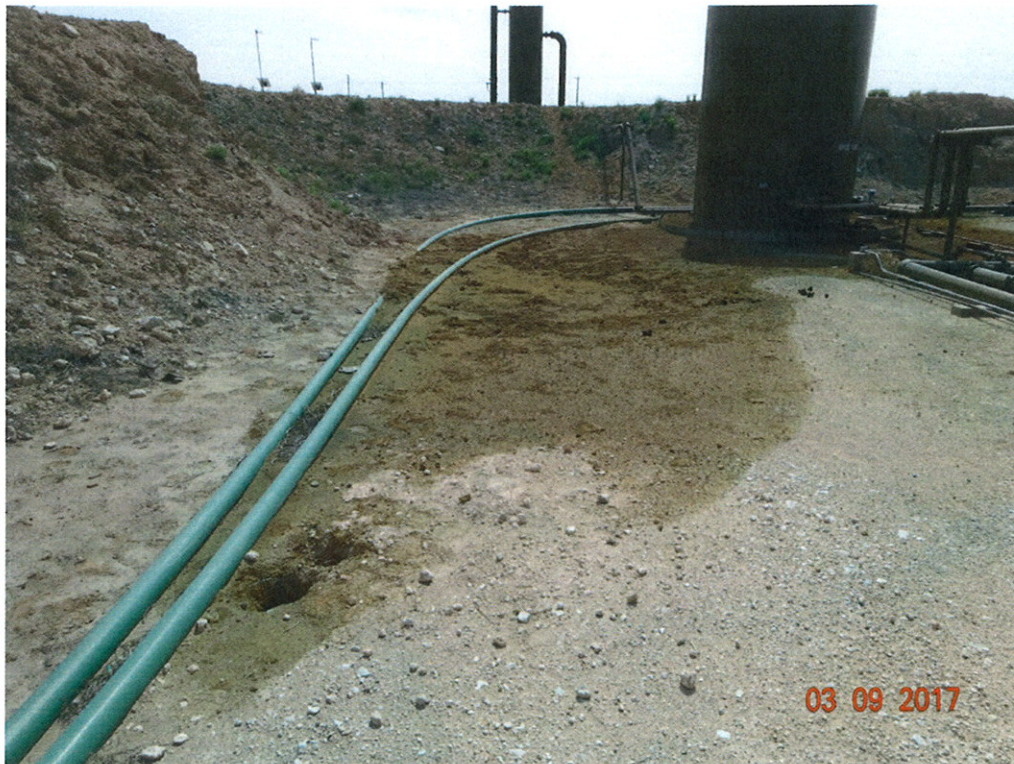
Spill Area Viewing South
