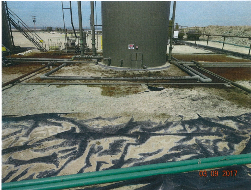
Spill Area Viewing North
