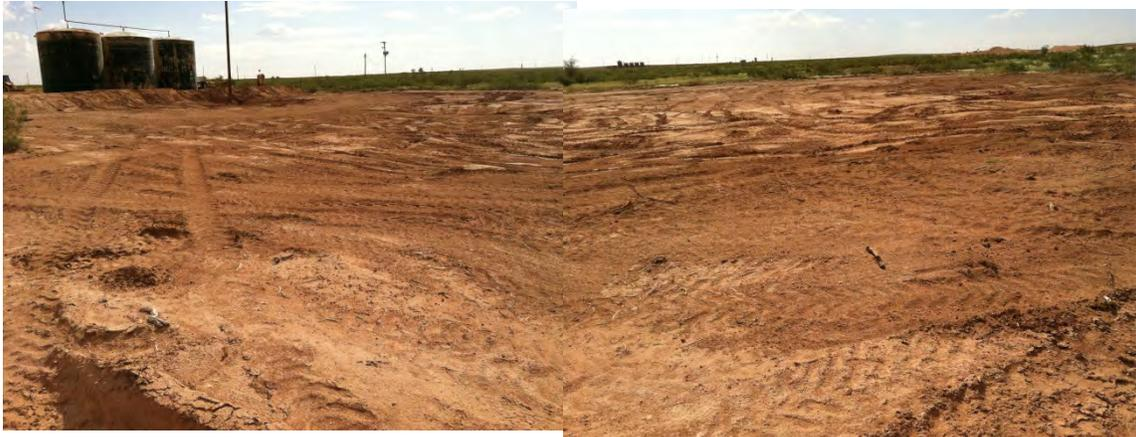
View to the northwest of release footprint after excavation of soil stained by hydrocarbons.
