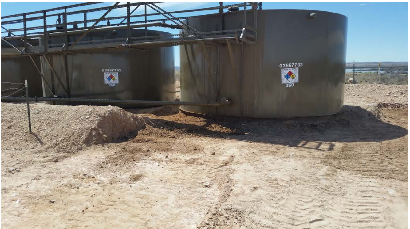
Firewall removed, affected soils mostly removed
