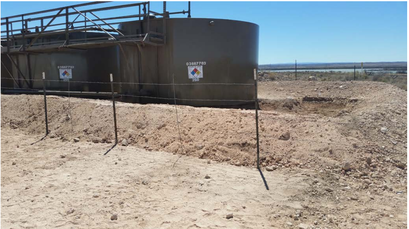
Firewall and fence replaced
