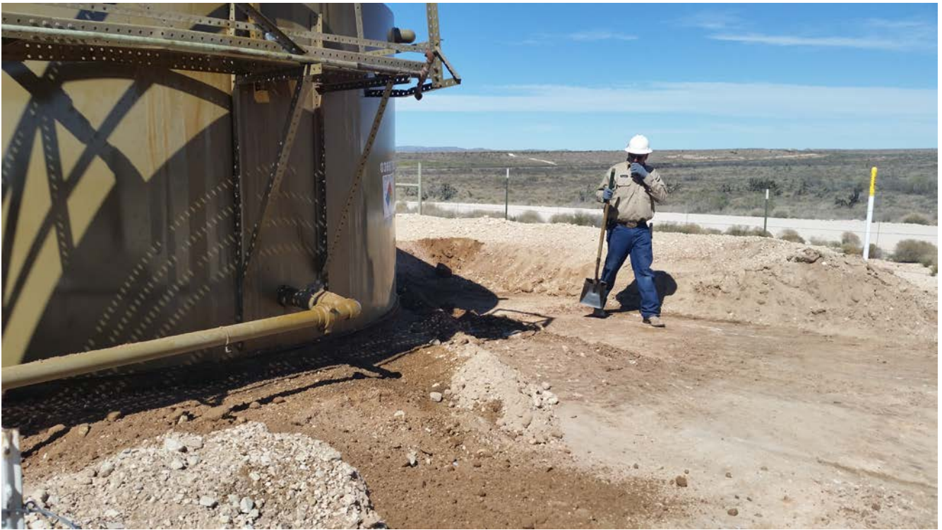
Firewall removed, affected soils mostly removed
