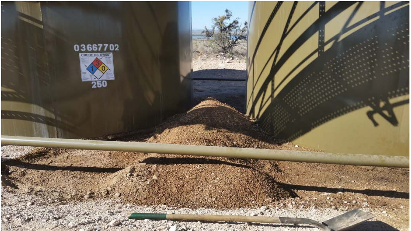
Removing affected soils
