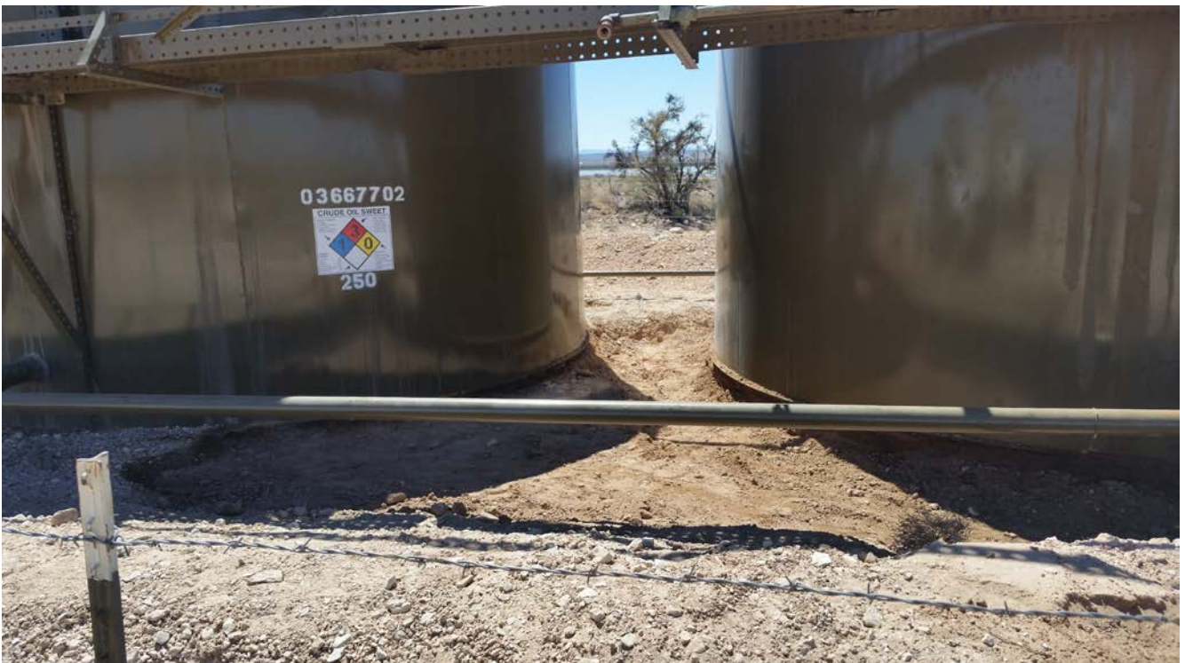
Excavated area prior to backfilling with new pea gravel
