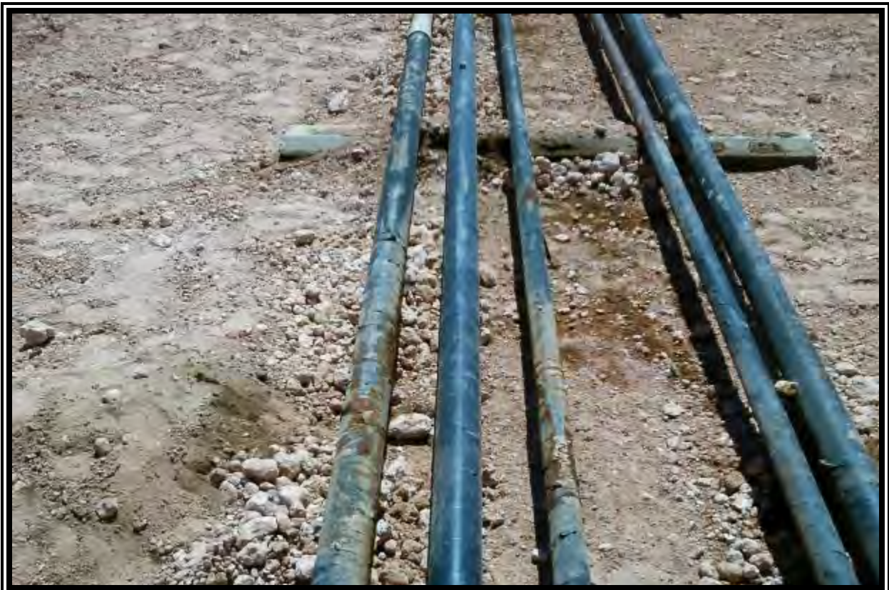
View of repaired line and initial remediation activities.
