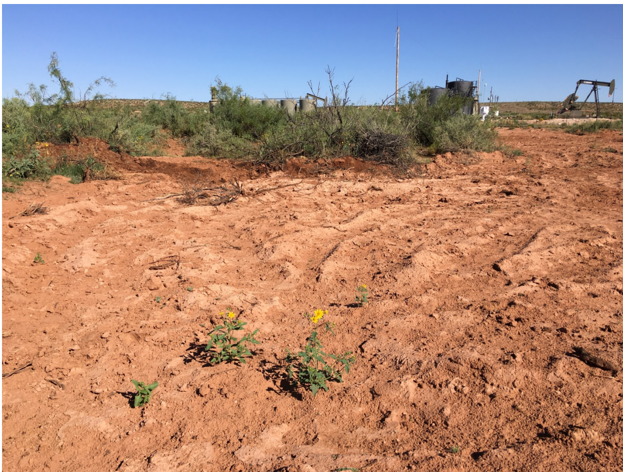
Figure 2 – Area of excavation near sampling location S7 with the BDU 21 in background. Note that volunteer vegetation is starting to grow in this area. About 18-inches of soil/sand was removed from this portion of the spill footprint.
