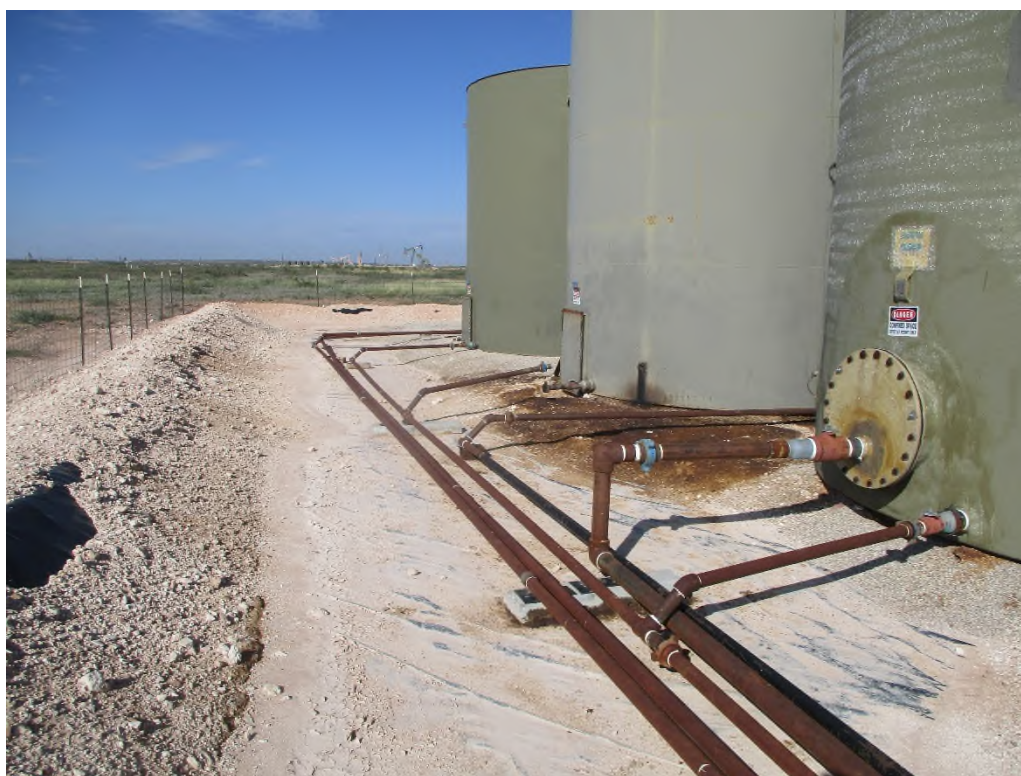
View West – Release Area
