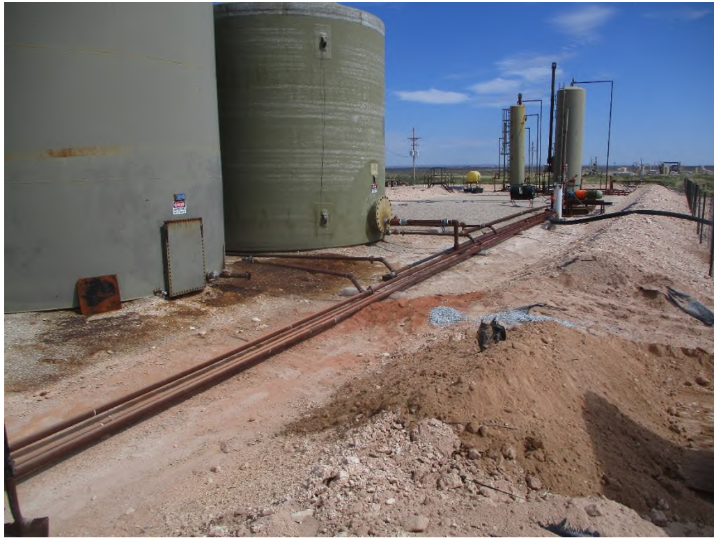
View Northeast – Area of BH-1
