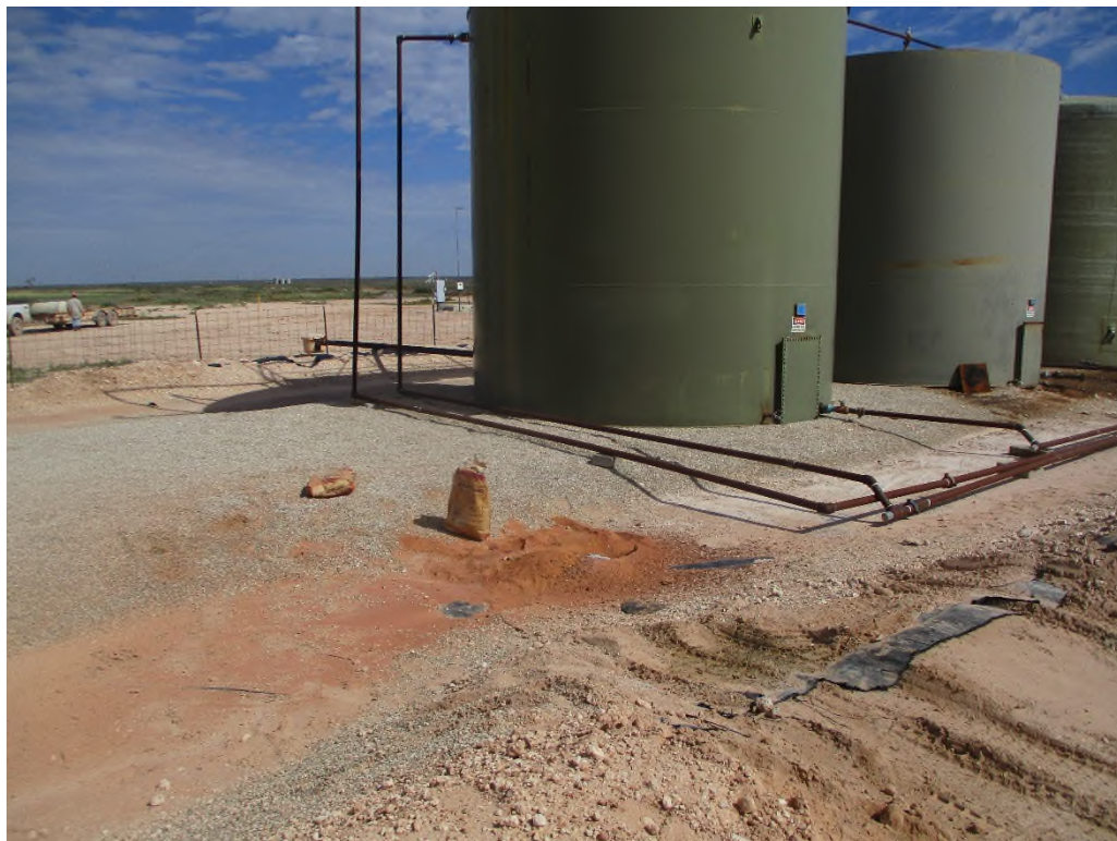
View North – Area of BH-2
