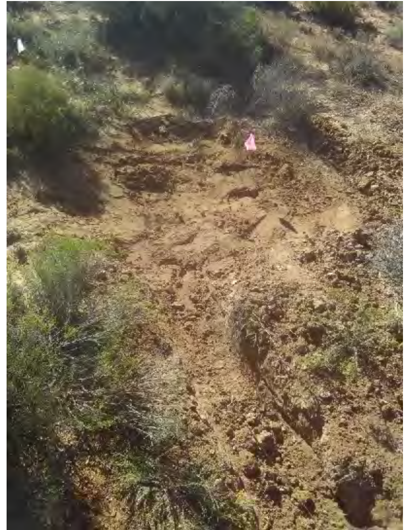
Sterling Silver 3 0005 – Excavation (Looking West)
