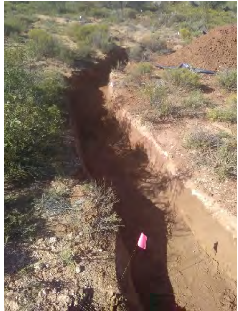
Sterling Silver 3 0005 – Excavation (Looking Northwest)
