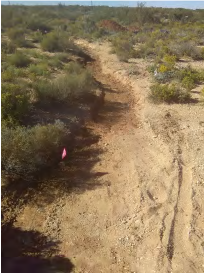
Sterling Silver 3 0005 – Excavation (Looking Northwest)
